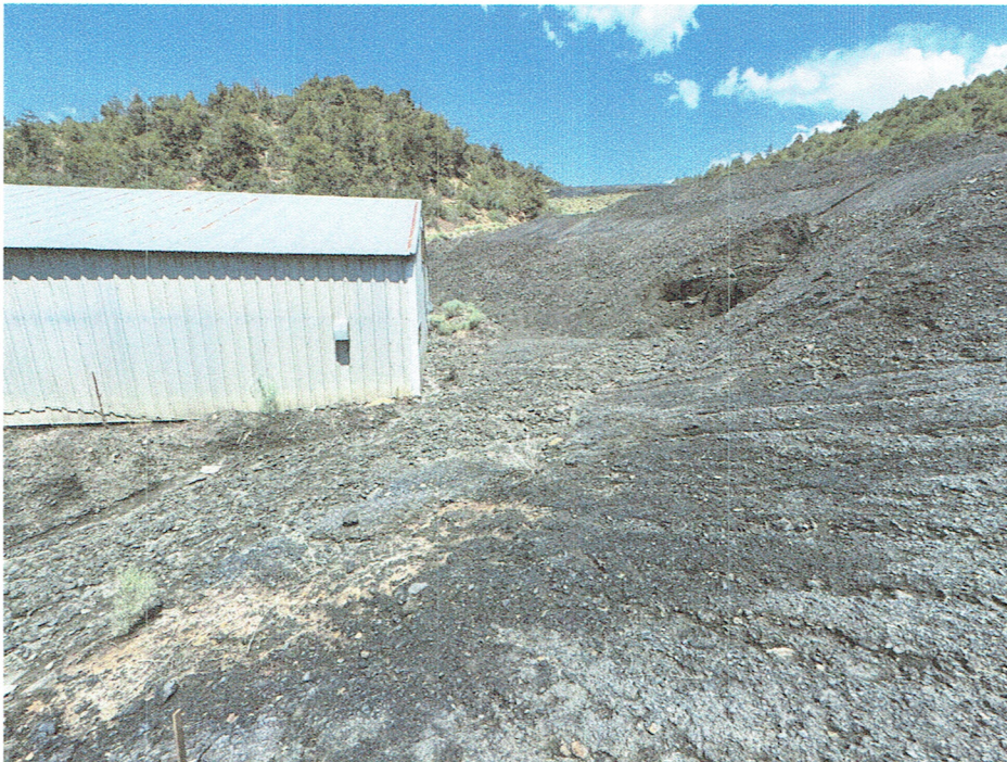
Pic. 4 – Erosion of face of lower waste pile south of old bath house.
