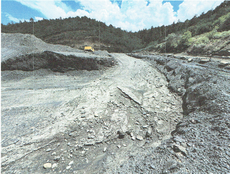
Pic. 3 – Erosion from surface runoff at equipment access of lower waste pile.
