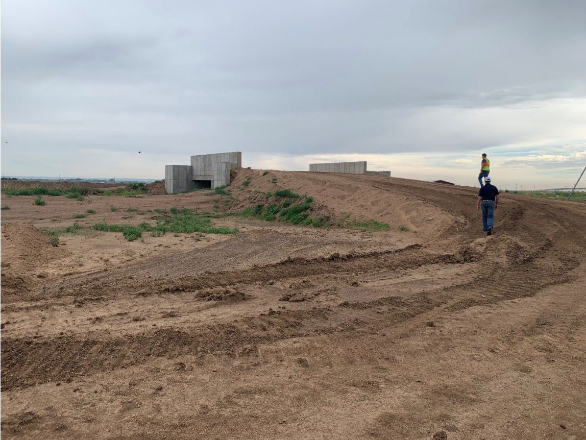
Photo 5 – Boxed culvert installed over the Western Mutual Ditch.
