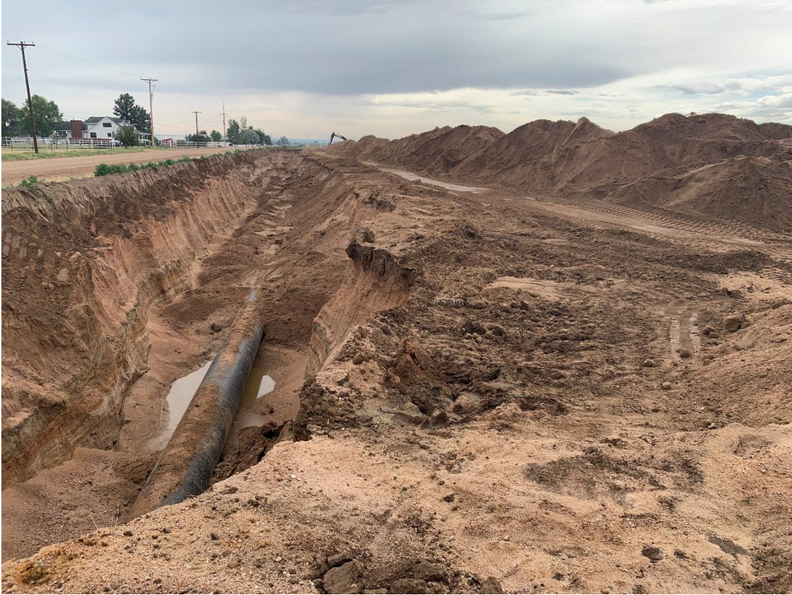
Photo 3 – Buried water pipeline on western boundary of proposed permit area.
