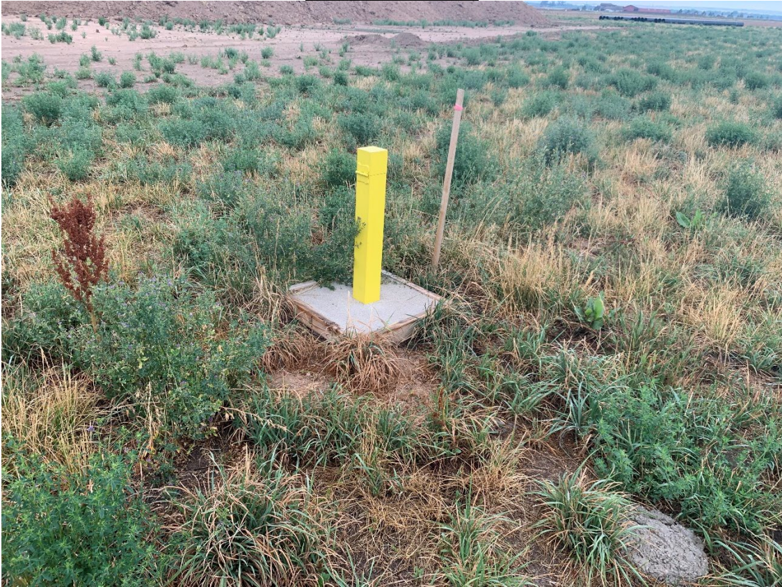
Photo 1 – Monitoring well MW-3 in the southeast corner.
