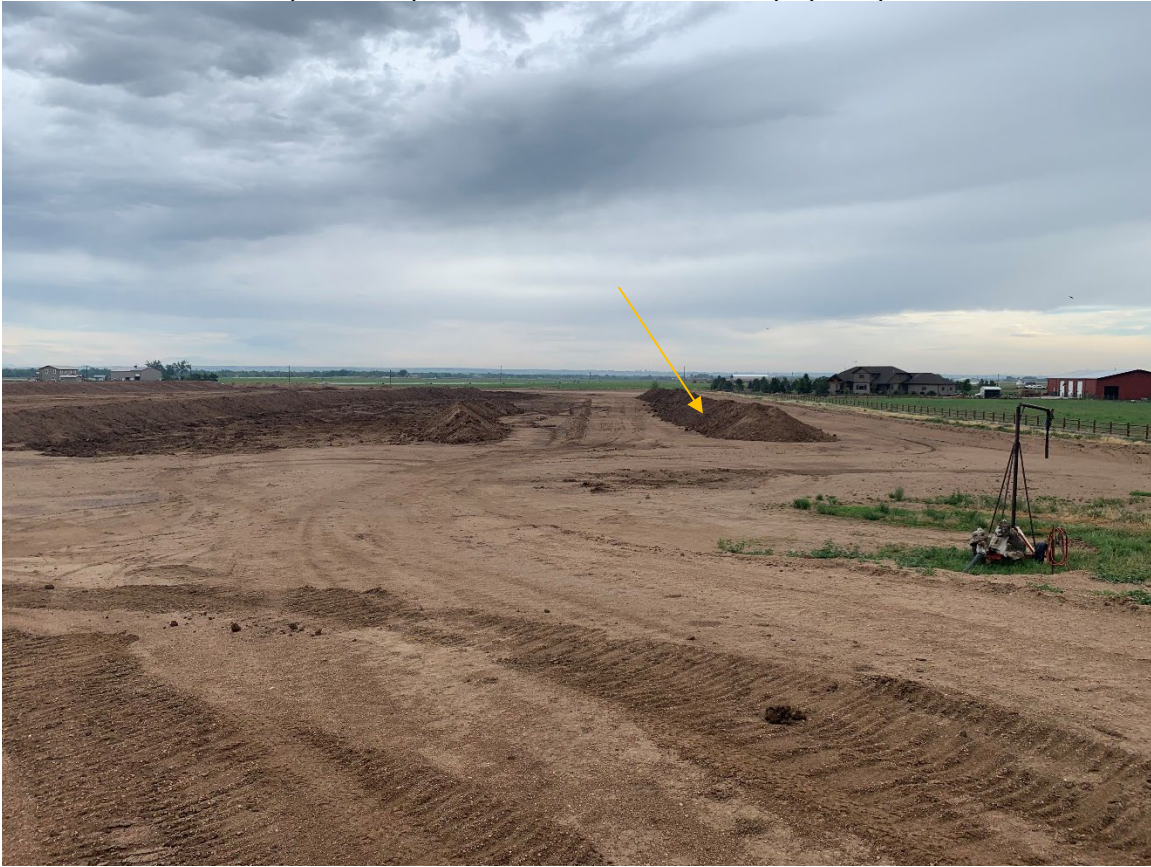
Photo 8 – Salvaged soil for slurry wall construction stacked in rows.
