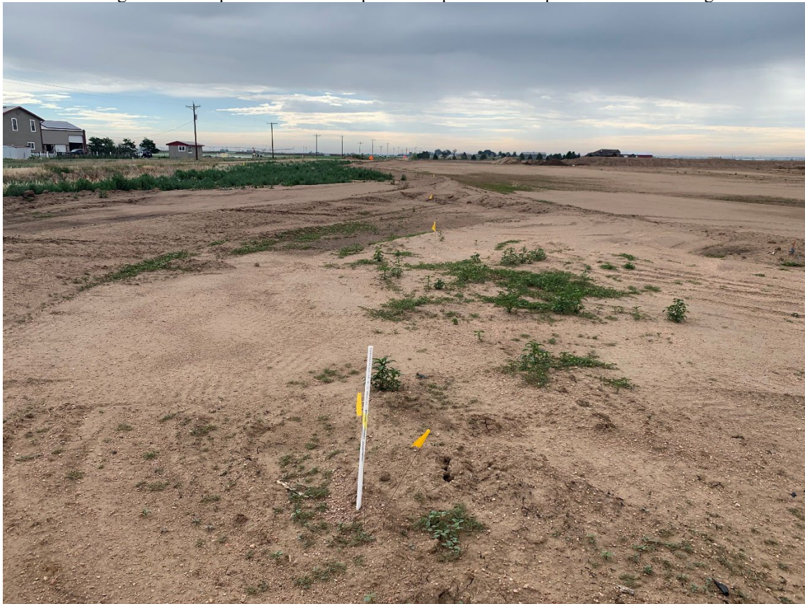
Photo 10 – Exiting gas lines were marked with yellow flags.
