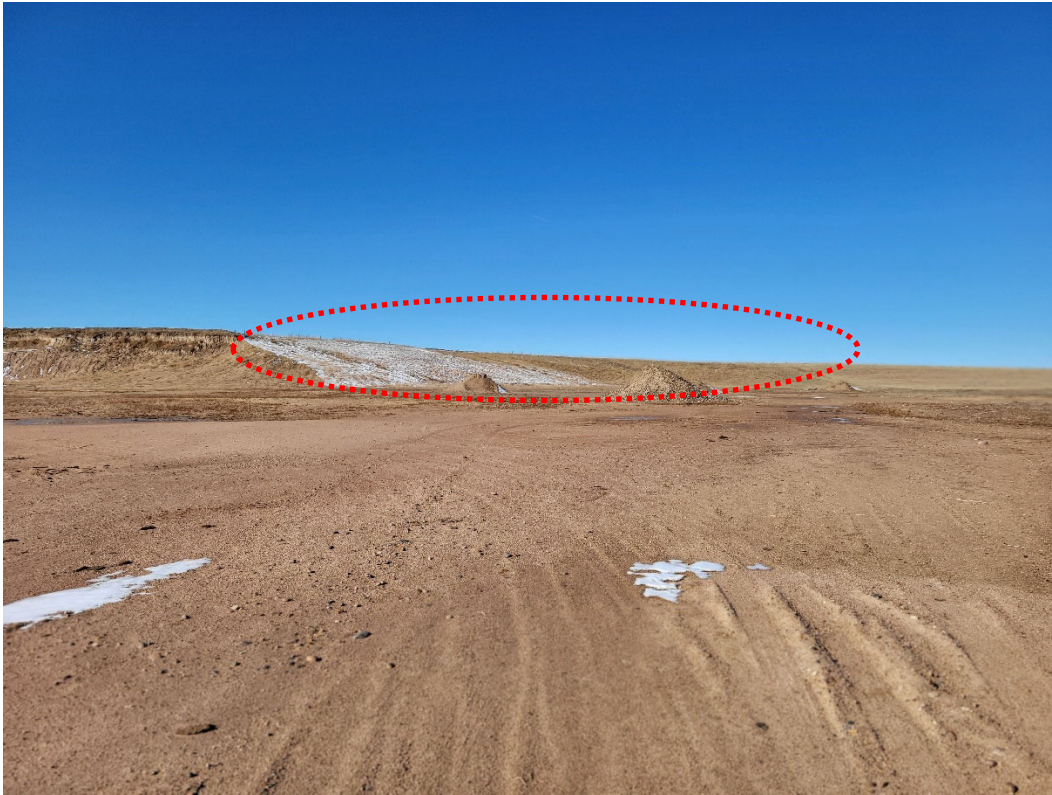
Photo 3: Looking west. Area circled topsoiled and seeded. Stockpiled material stored on the pit floor.
