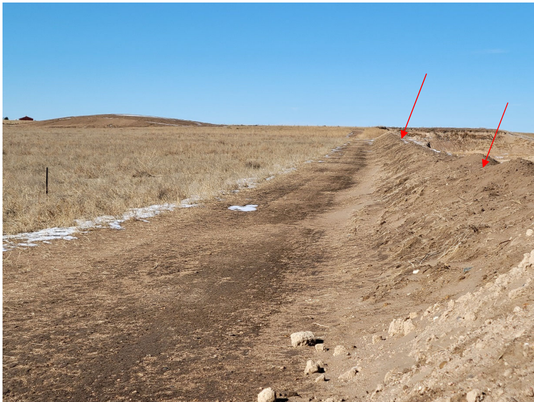
Photo 4: Looking west above the highwall on the south side. Overburden stored in berms (arrows) for future use in reclamation.
