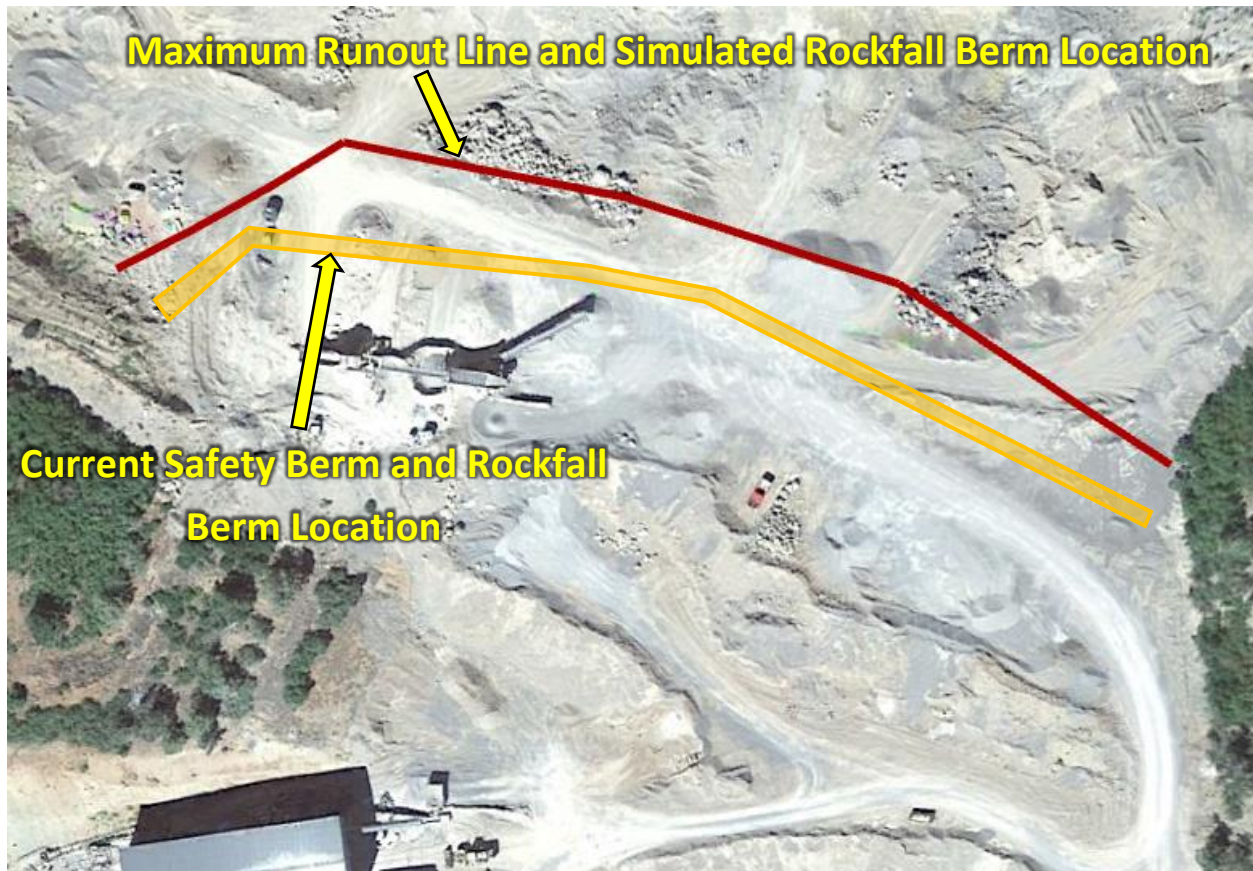
Figure 3 – Placement of Rockfall Berm on North Edge of Access Area
