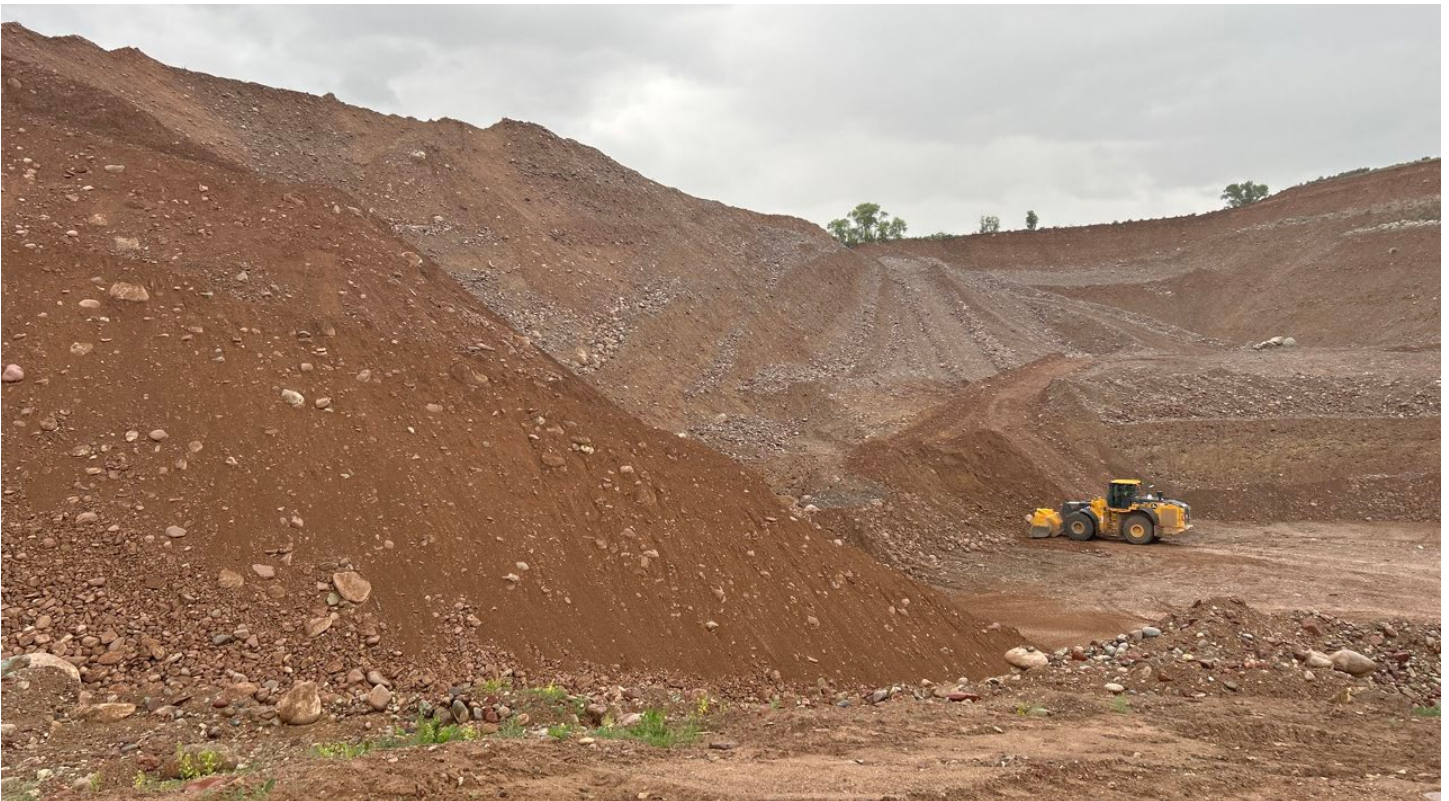
Figure 7: Active highwall. No blasting. Dozer pushes material down to loader. Pont 309
