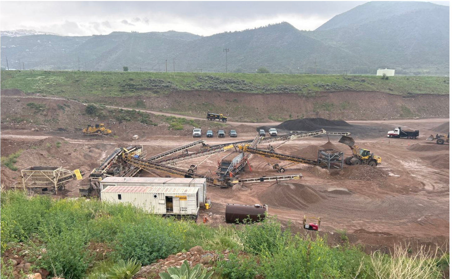
Figure 10: Crushing/screening operations in progress
