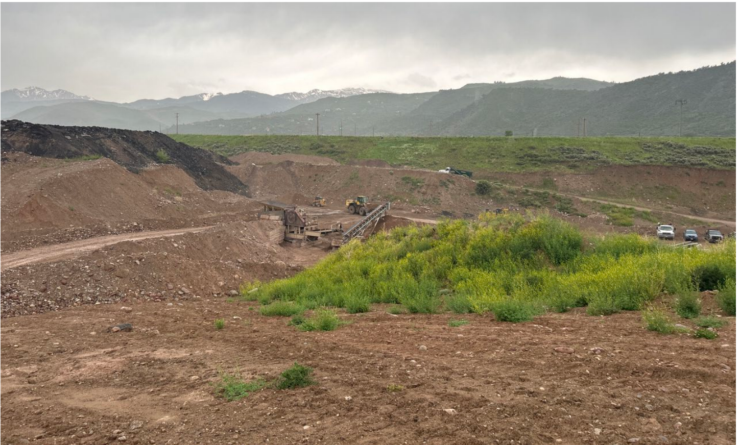
Figure 9: Loader route to crusher. Point 309
