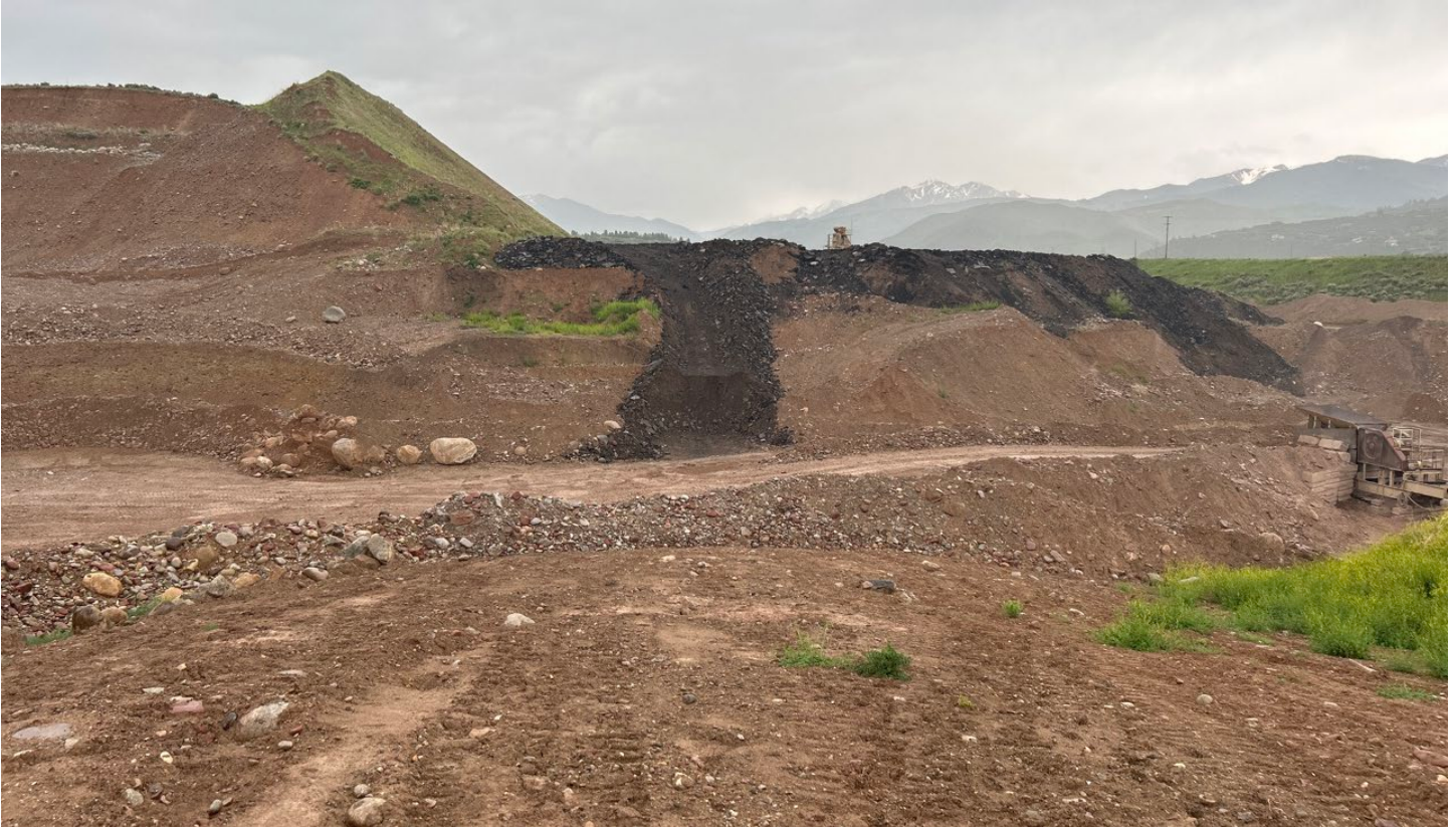
Figure 8: Dozer push area for asphalt. Point 309
