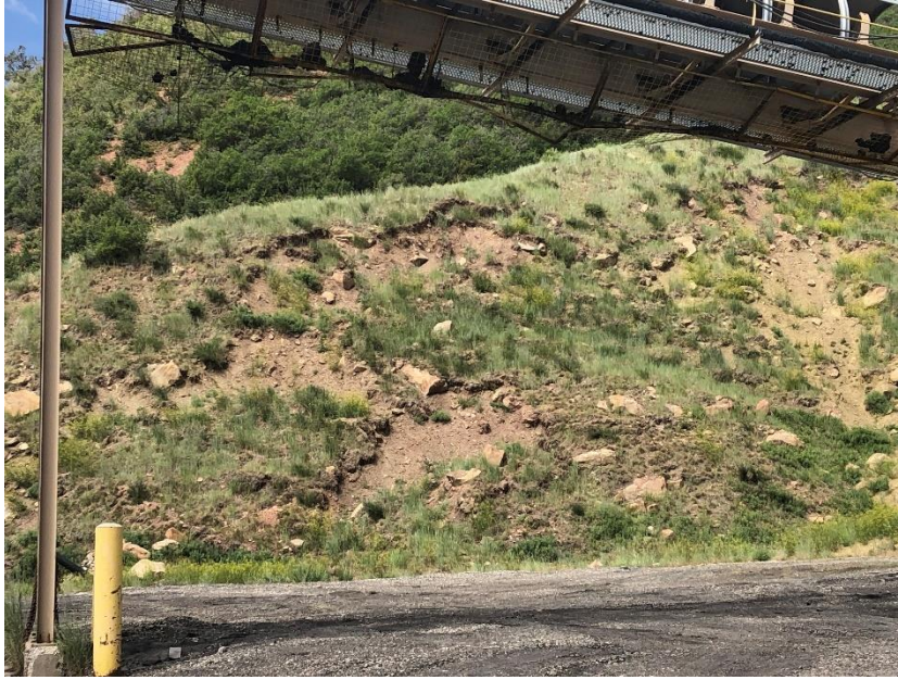
Slump at B Portal bench
