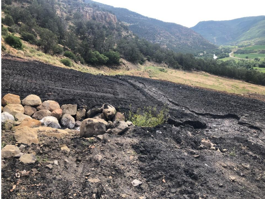
Ditch on Gob Pile #2 that needs to be constructed
