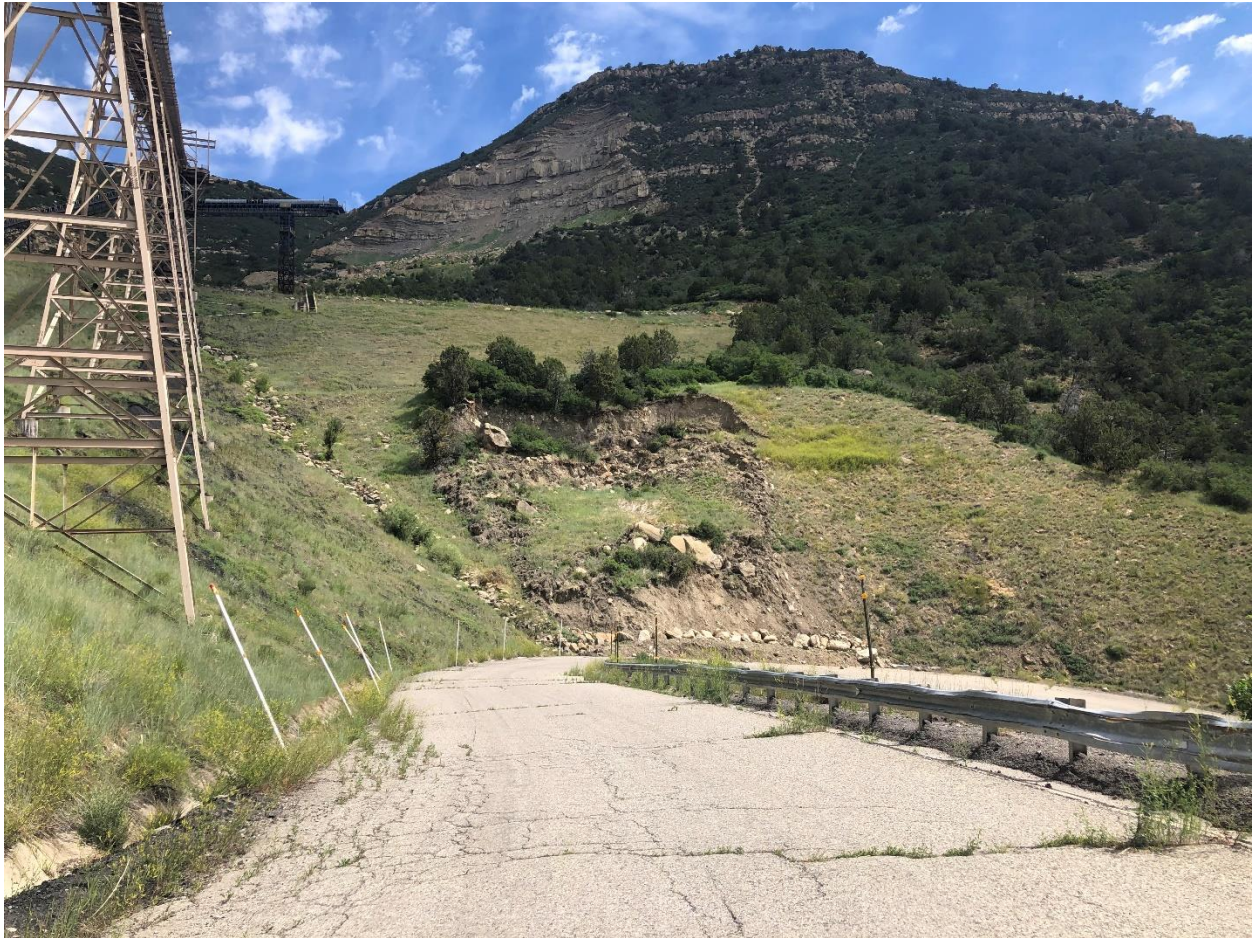
Slide at Curve 10 – appears to still be moving
