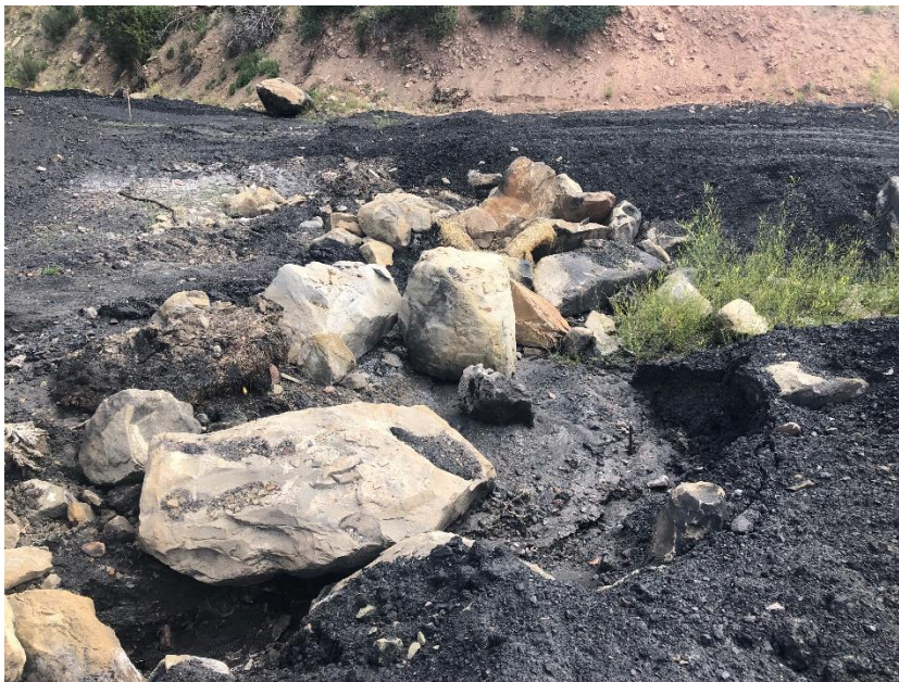
Disassembled BMPs on Gob Pile #2 – need to be reassembled when practical
