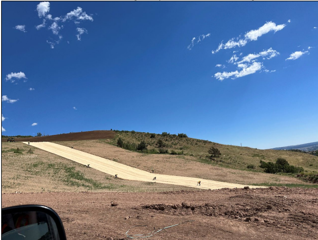
Photo 3: Erosion control matting was being placed on a northeastern slope where erosion rills were present.
