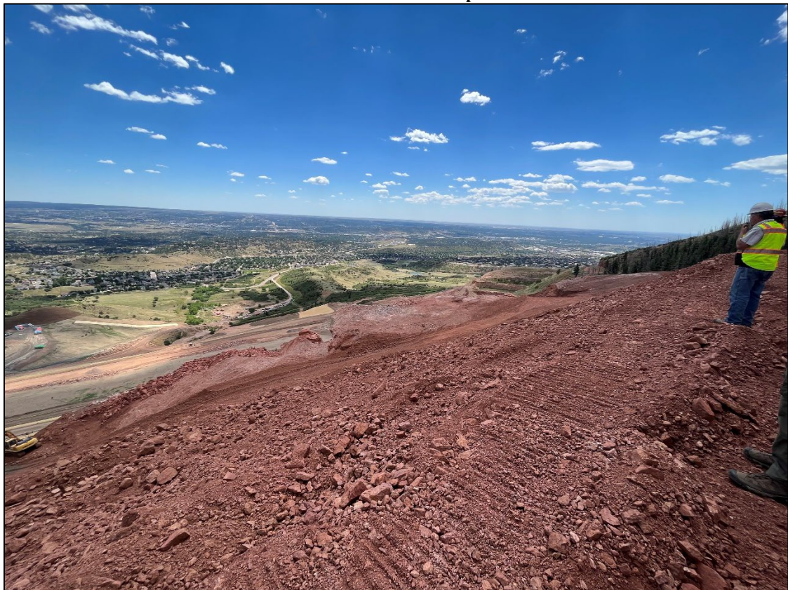
Photo 9: View of the BFR, the southern extent is begin filled in to grade, rocky material has been left below the BFR to serve as wildlife habitat.
