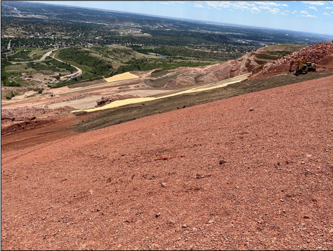
Photo 10: View of the tension crack slope, topsoiling has begun on the southern portion of this slope.
