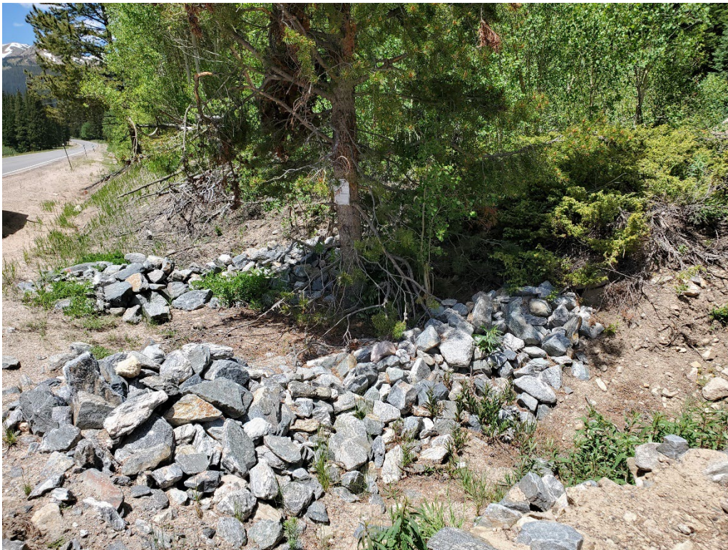
Photo 4: Looking west at a series of rock check dams along the entrance to the access road.
