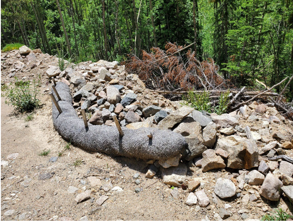
Photo 7: Looking north-east at a check dam and straw wattle along the access road.
