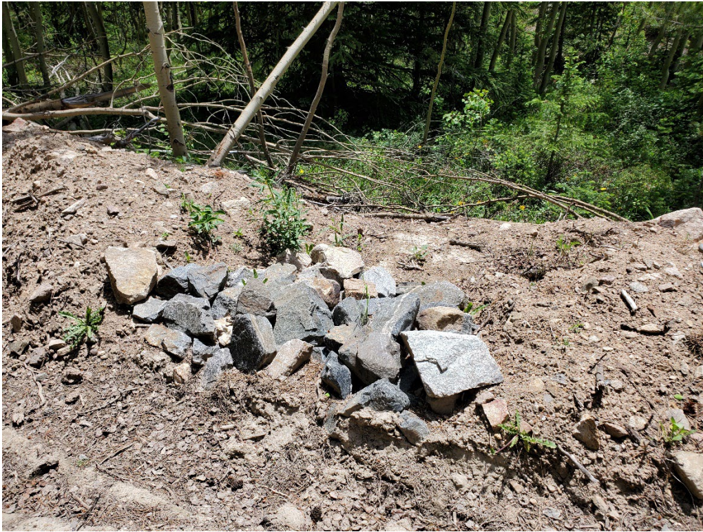
Photo 5: Looking north-east at a check dam along the access road.
