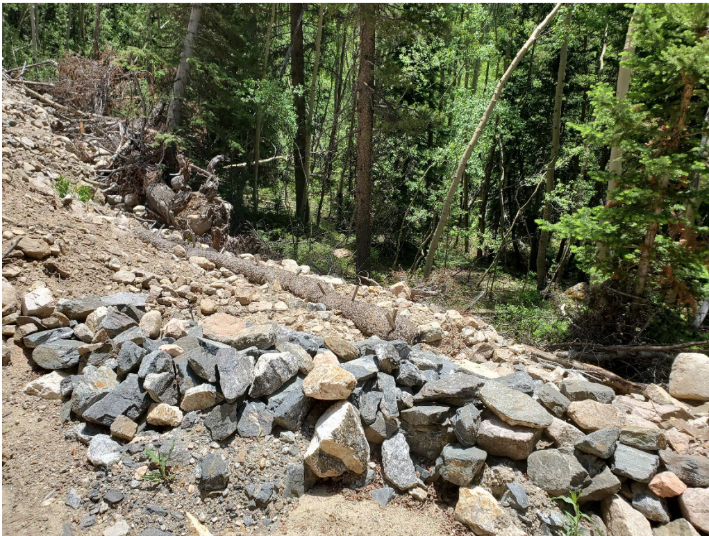
Photo 6: Looking north-east at a check dam along the access road.
