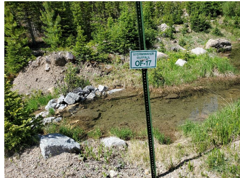
Photo 27: Looking southwest at check dams along No Name Gulch, south of OF-17.
