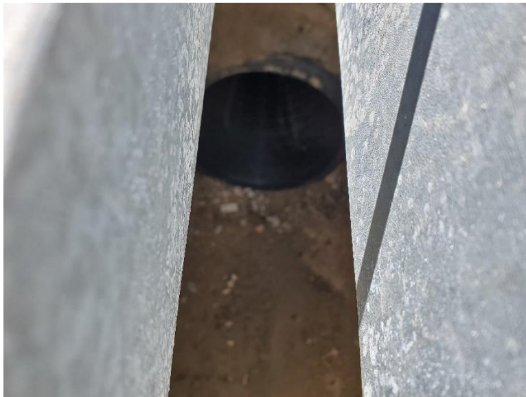
Photo 29: Looking into the grate of the box culvert. The culvert is free of obstructions.
