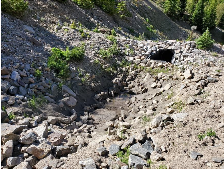
Photo 25: Looking south at the rip-rapped drainage basin at OF-15.
