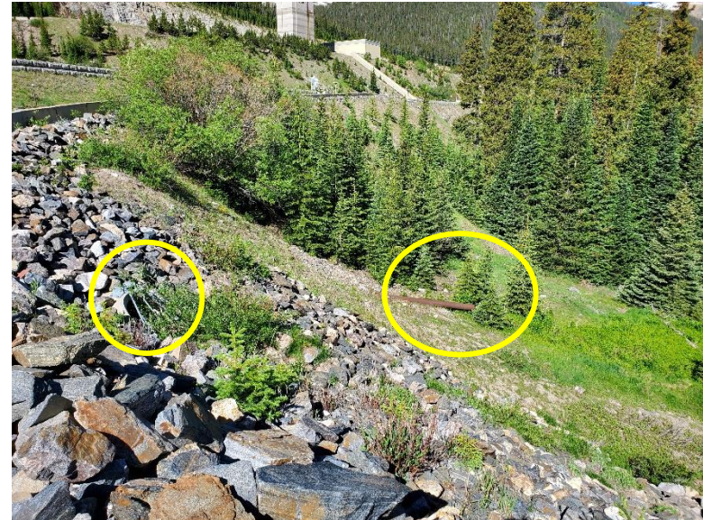
Photo 19: Circled are two drainage pipes (one box culvert one metal pipe), discharging onto the rip-rapped slope leading to OF-9.
