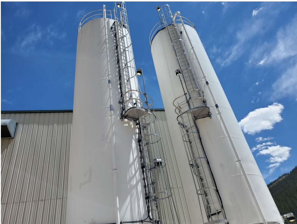
Photo 2: Lime silos located on the south side of the URAD water treatment plant.
