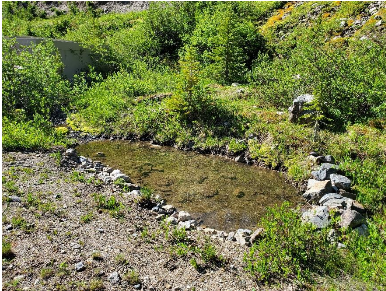
Photo 18: Rip-rapped drainage basin located upslope and south of OF-9.
