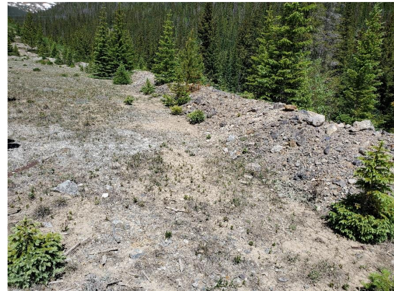
Photo 22: Looking west along one of the perimeter berms. Photo shows evidence of standing water (mudcracks) retained by the berms and leading to OF-12.
