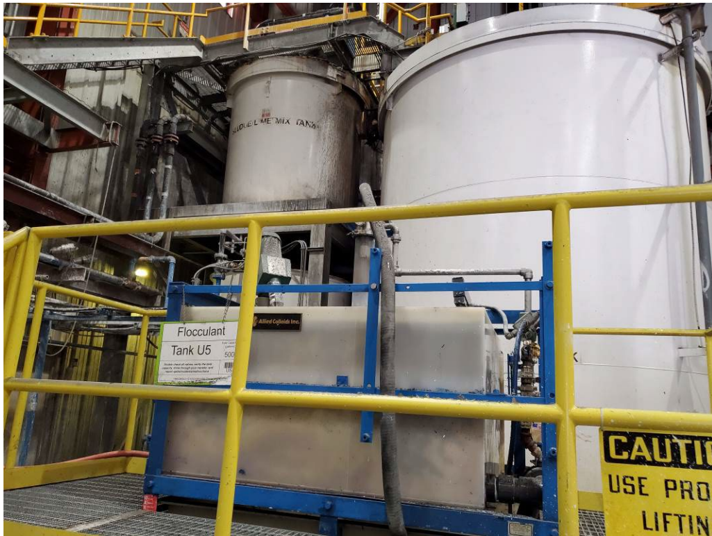
Photo 3: Floculant storage tank located within the URAD water treatment plant.
