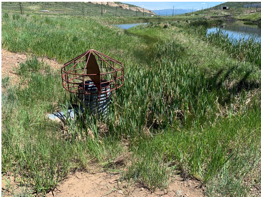
Photo 7 – Pond E discharge point needs to have cattails cleared.
