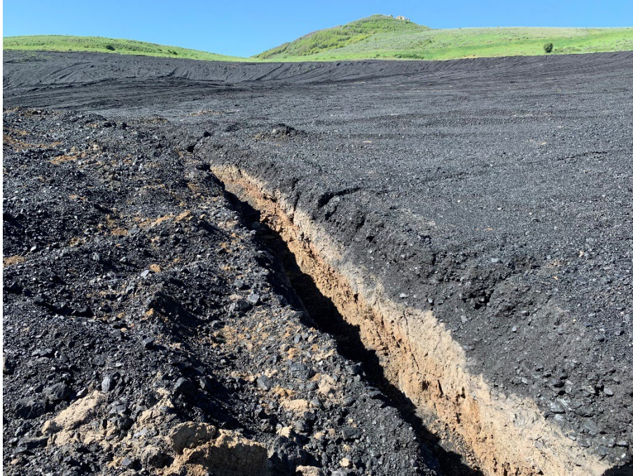
Photo 13 – French Drain trench under the BOB pile
