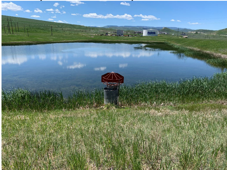
Photo 10 – Pond G primary spillway structure
