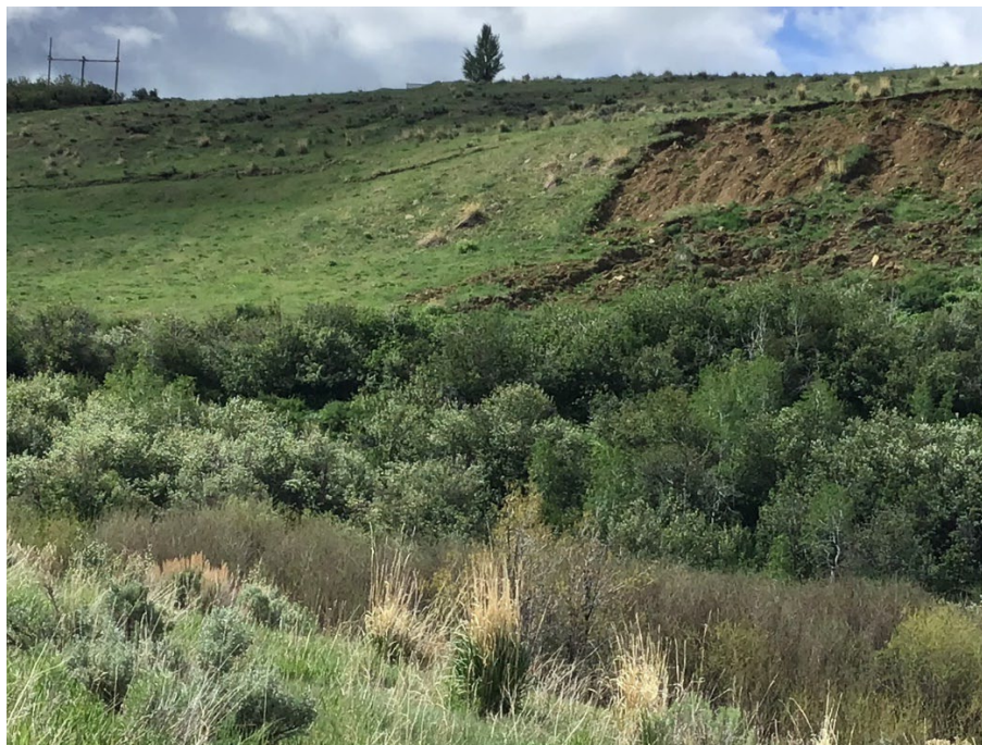
Photo 2: Pond 6 spring 2023 slump with crack going across the slope.
