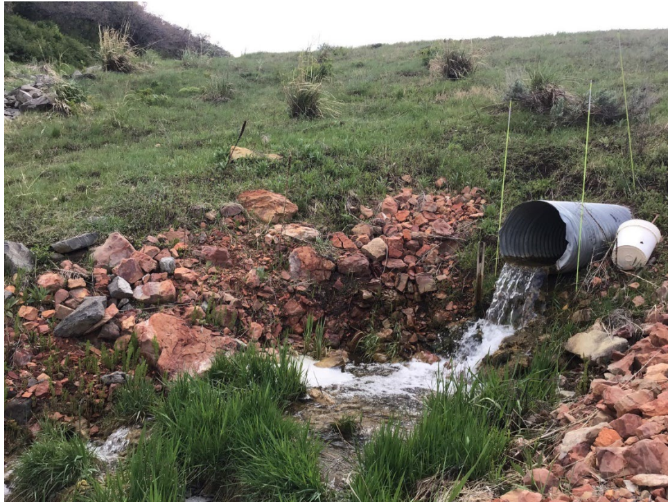
Photo 9: Pond 16 discharge culvert.
