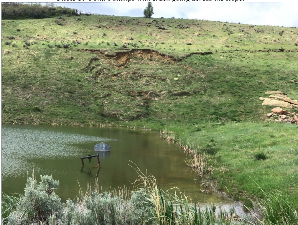
Photo 4: Pond 6 old slump with crack going across the slope.
