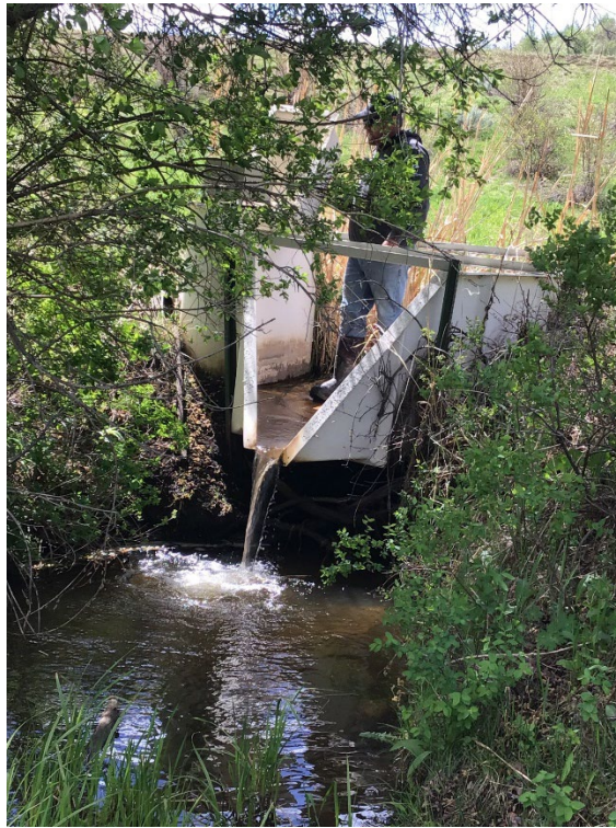
Photo 13: Pond 17 flume. Grasses at flume entrance require removal.
