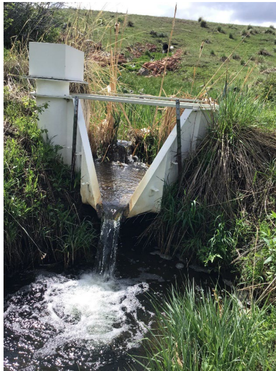
Photo 11: Pond 16 flume, vegetation requires clearing.
