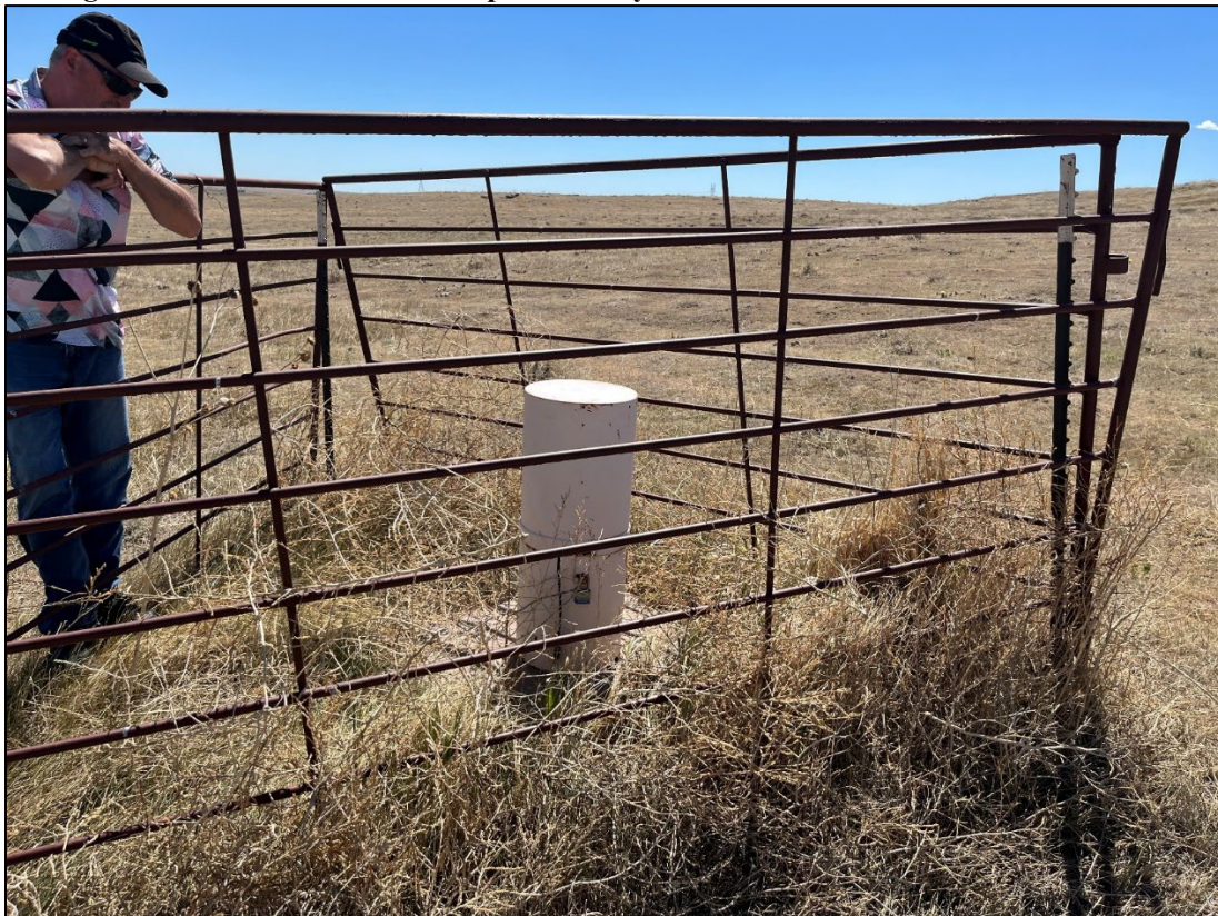
Figure 2: Wells are protected by cattle guards.
