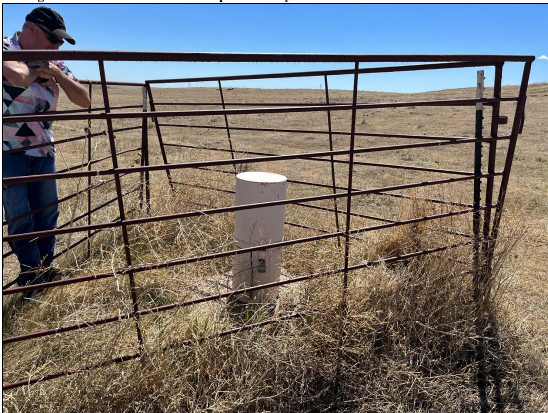
Figure 2: Wells are protected by cattle guards.
