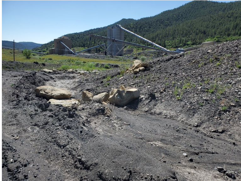
Photo 3: First check dam, located on the north-east side of DWDA #2.
