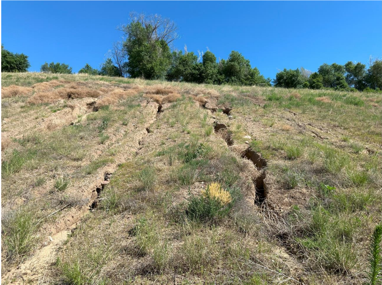
Photo 5. Erosion gullies in central area of buttress
