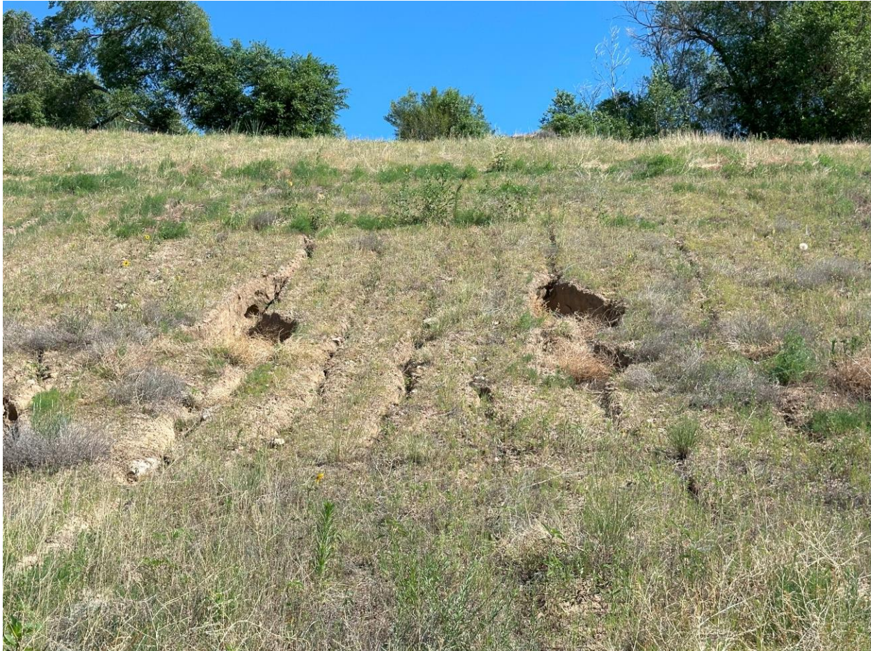
Photo 2. Erosion gullies in western area of buttress
