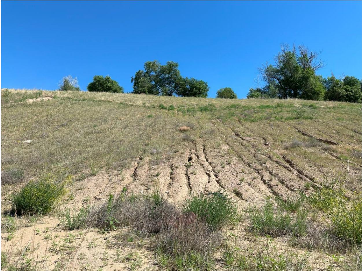
Photo 3. Erosion gullies in western area of buttress
