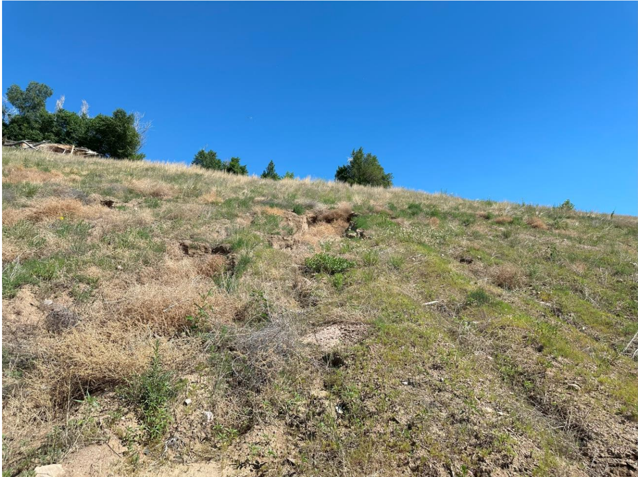
Photo 4. Erosion gully in eastern portion of buttress
