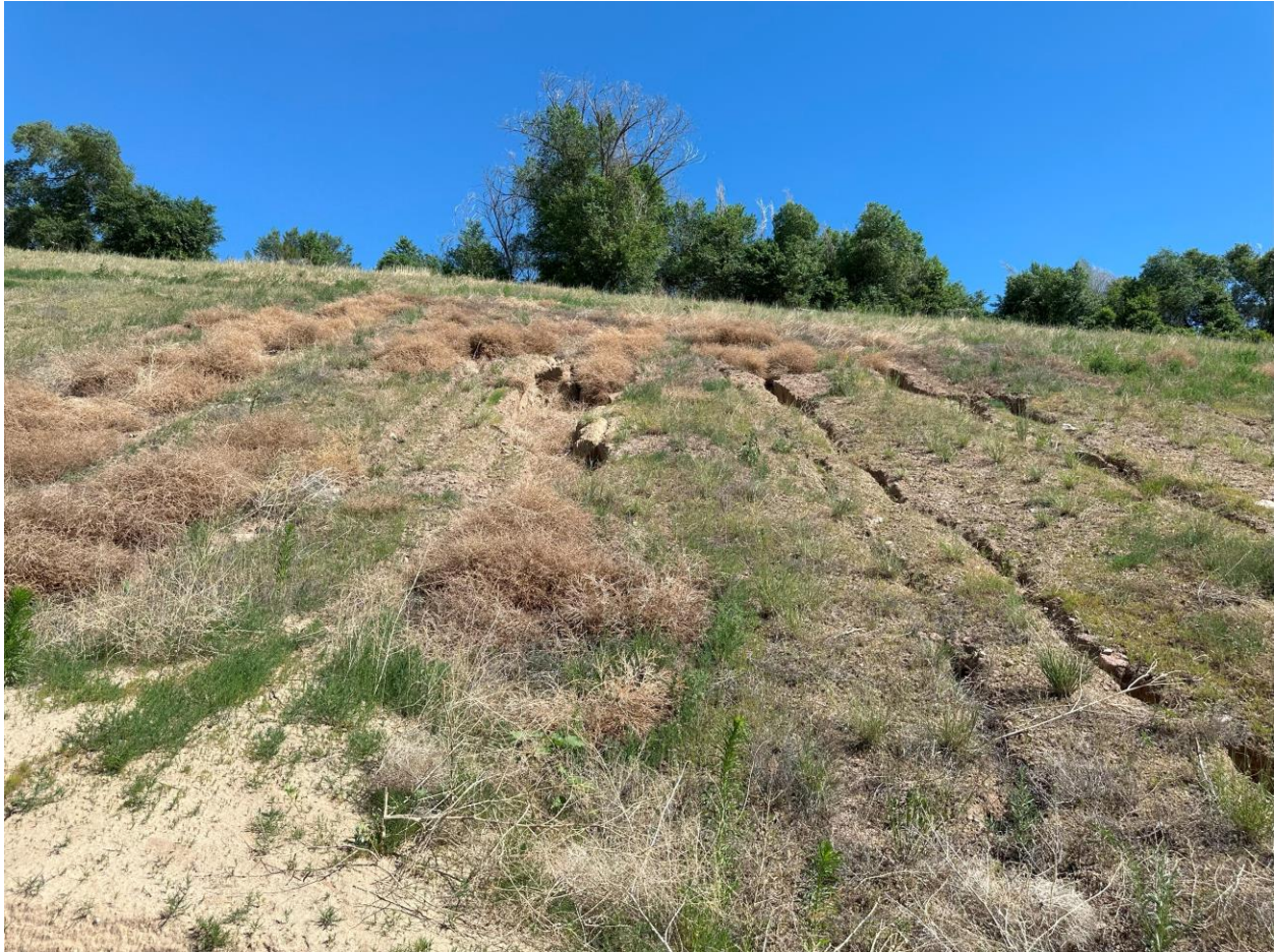
Photo 6. Erosion gullies in central area of buttress
