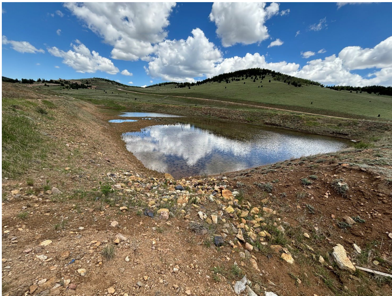
Photograph 3: View of the EMP-17 prior to pumping. Photo taken 4/10/2024 at approximately 10:00 MDT.
