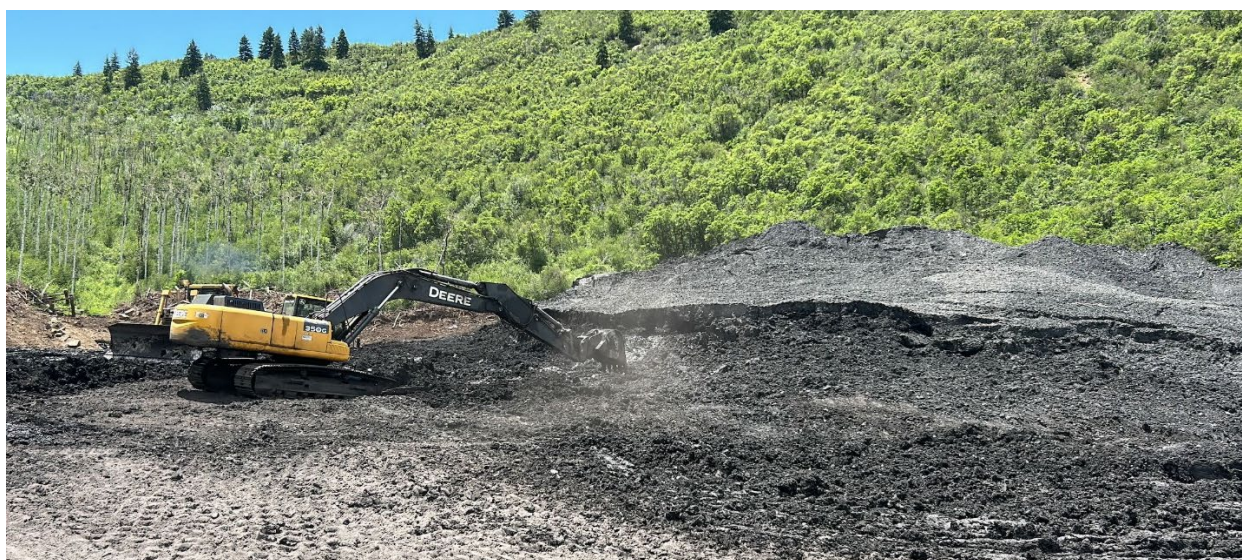
Figure 5: Excavator reaching for wet material on RPEE
