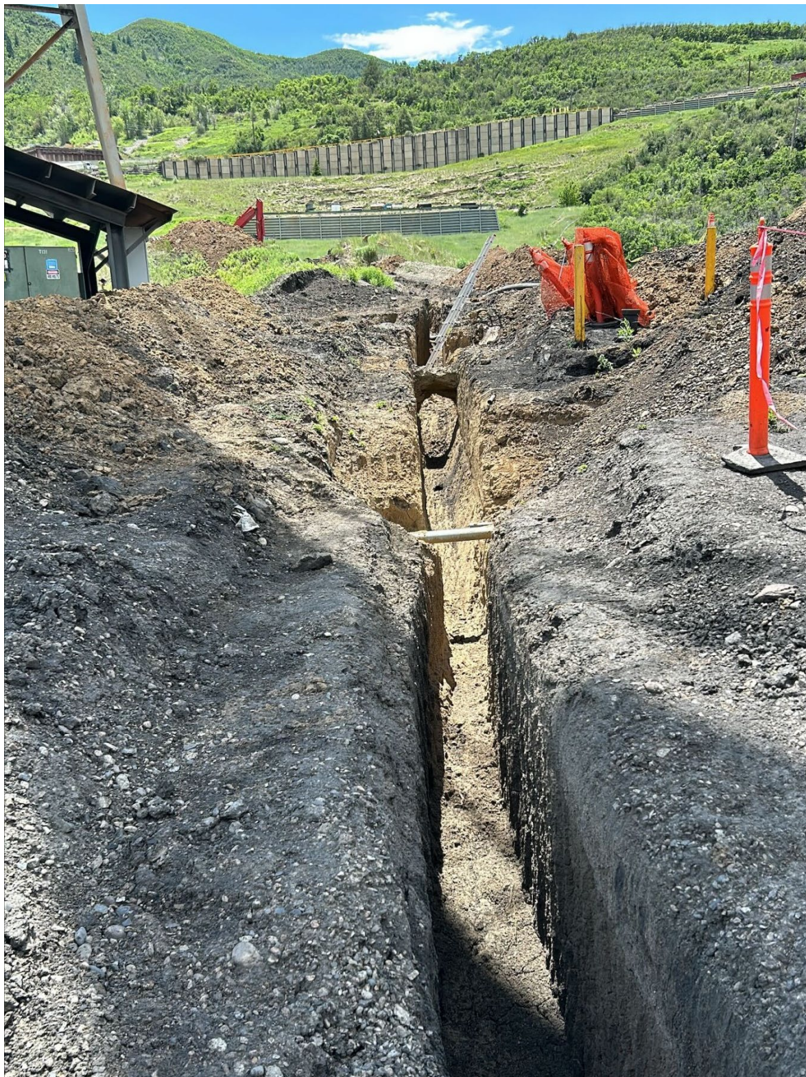
Figure 11: Upper end of trench for western BCN pipeline segment
