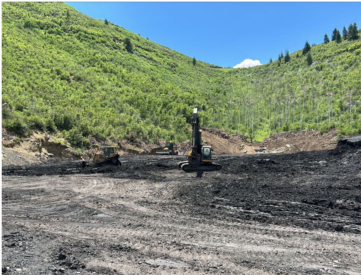
Figure 4: Excavator, dozer and sheep's foot compactor working on RPEE
