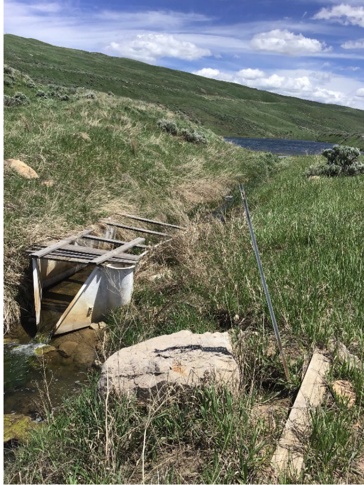
Photo 2: Flume at Pone 2, requiring replacement.
