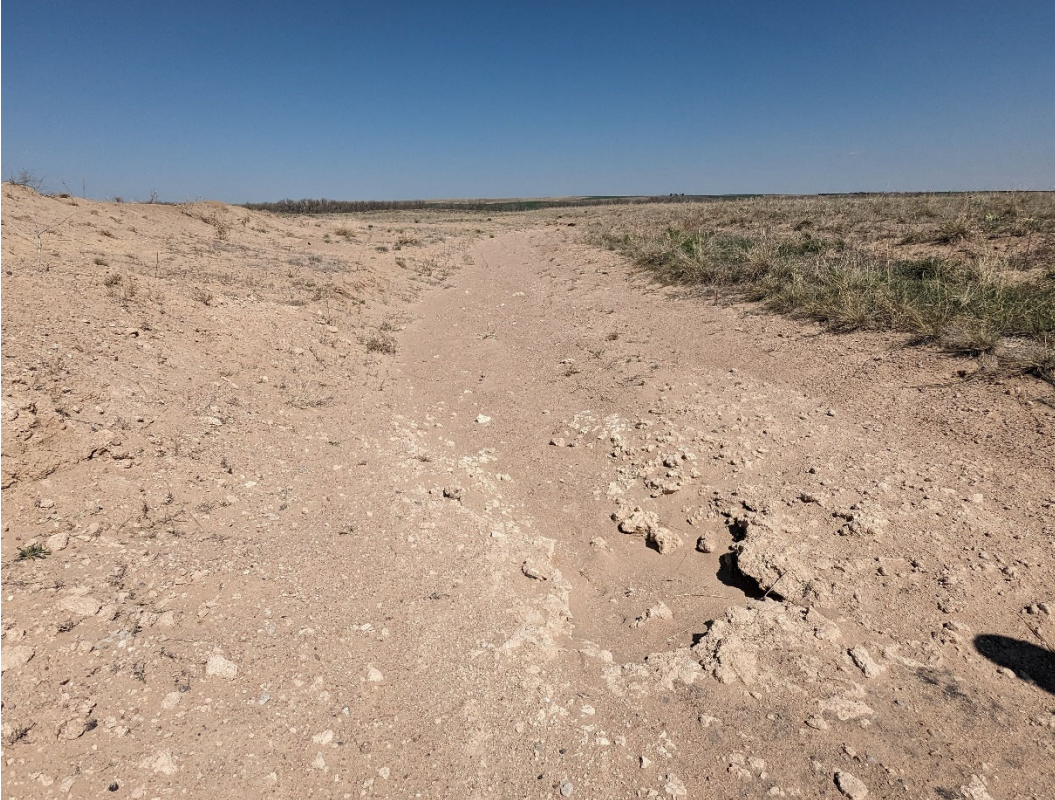
Photo 7: Runoff channel developing in the northwestern corner of the pit area. The Operator should install a berm and straw bales in this area to prevent sediment from leaving the pit during rain events.
