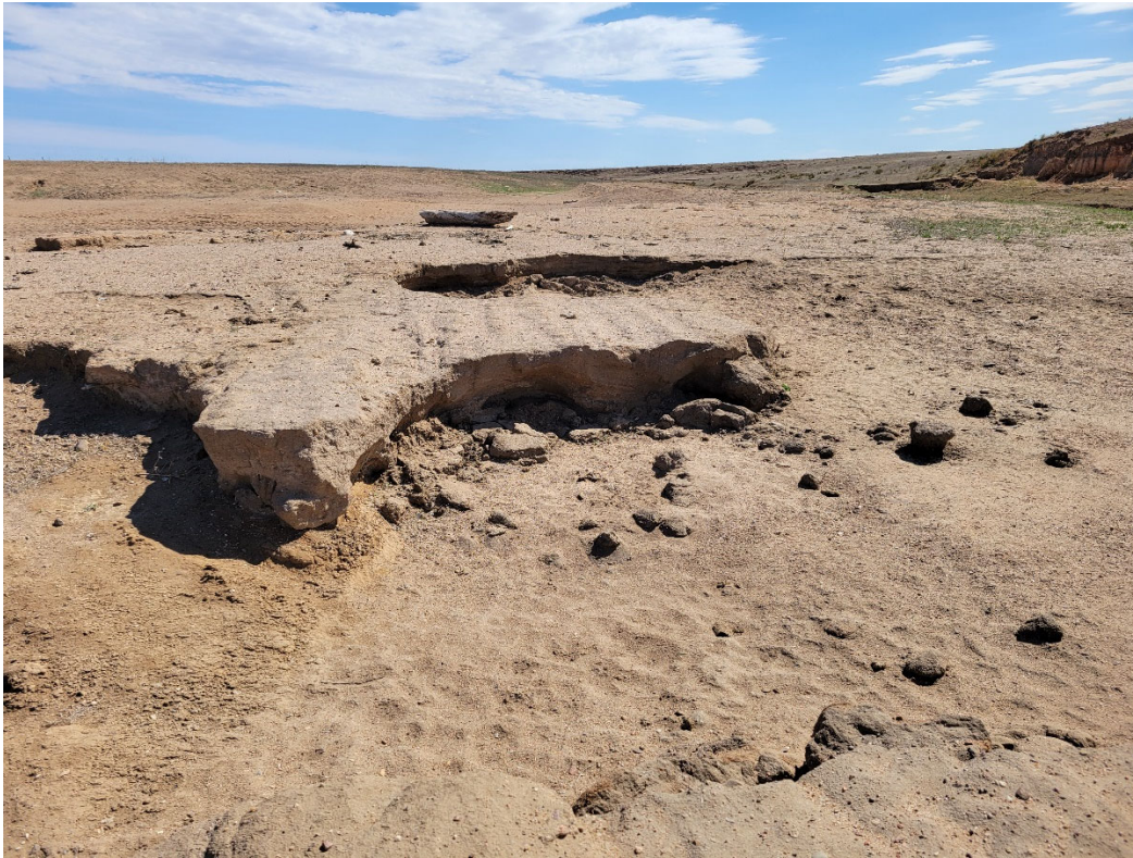
Photo 5: Entrance to the pit where the creek eroded the haul road.
