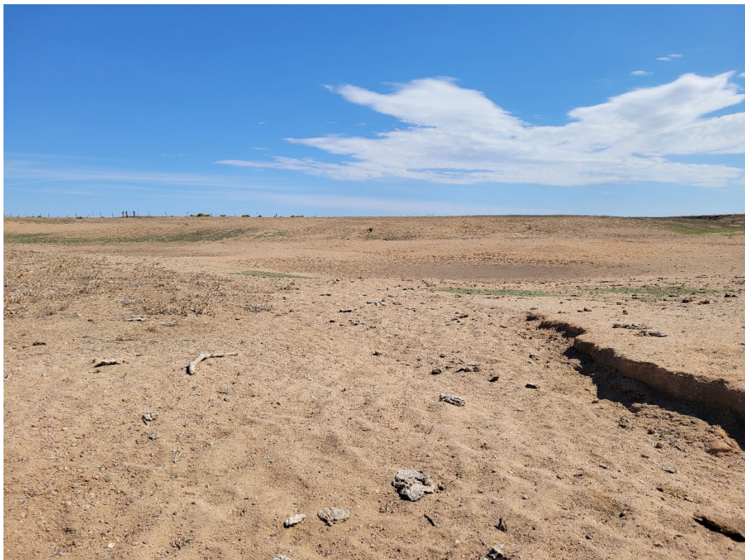
Photo 2: View looking northeast from the entrance to the pit. Slopes are graded 3H1:1V or shallower around the pit.
