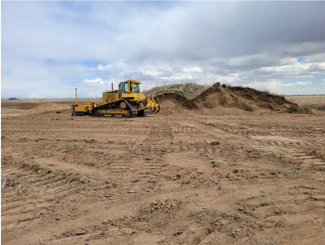
Photo 3: Dozer moving topsoil from top of pit to reclaimed slopes and relocated storage location at the bottom of pit.
