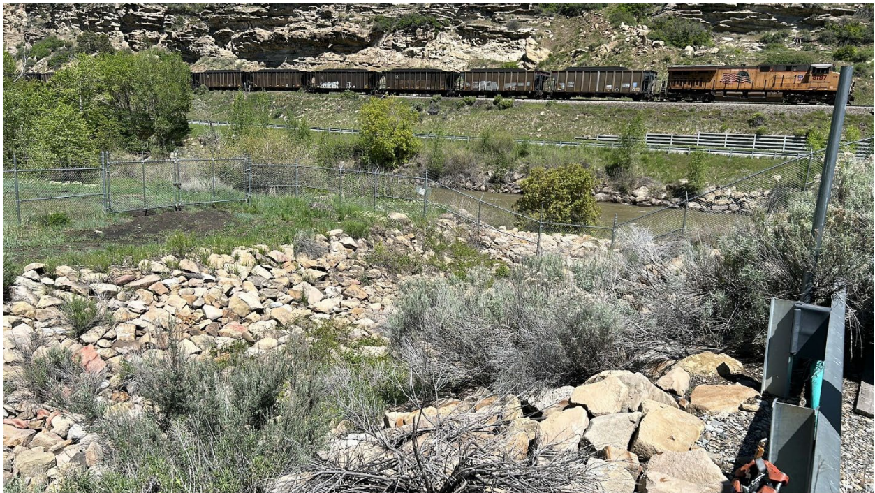
Figure 15: MB5E pond emergency spillway
