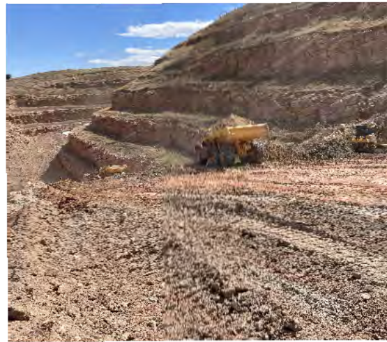
6. PLACING COMPACTED FILL ON BUTTRESS.
