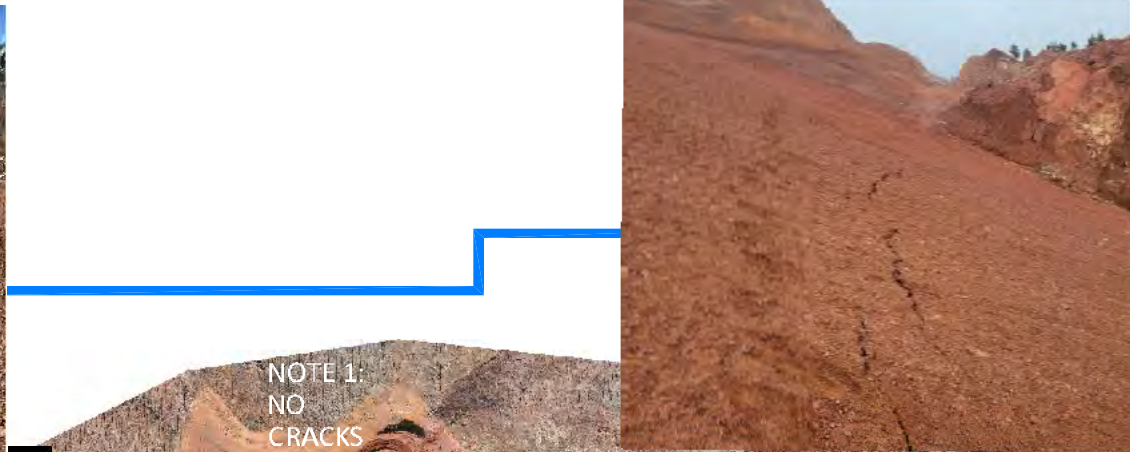
4. CRACKING ON UPPER FILL SLOPE.
