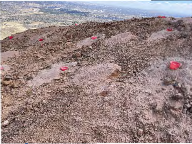
3. BLASTING PREPARATION ON SOUTH PEAK.
