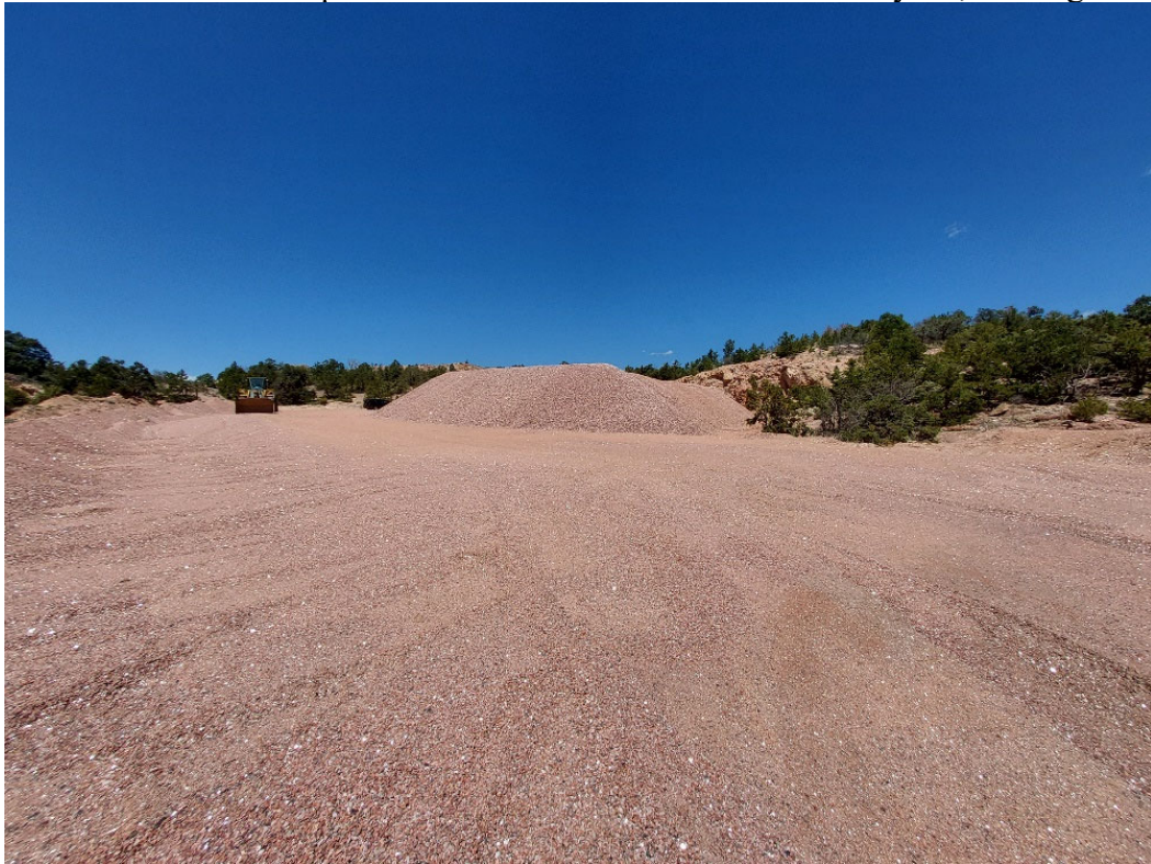
Photo #8: IMC-3 area, southeast of the Ruby Pit, looking north. The area is backfilled and graded; the stockpile of product material can be seen.
