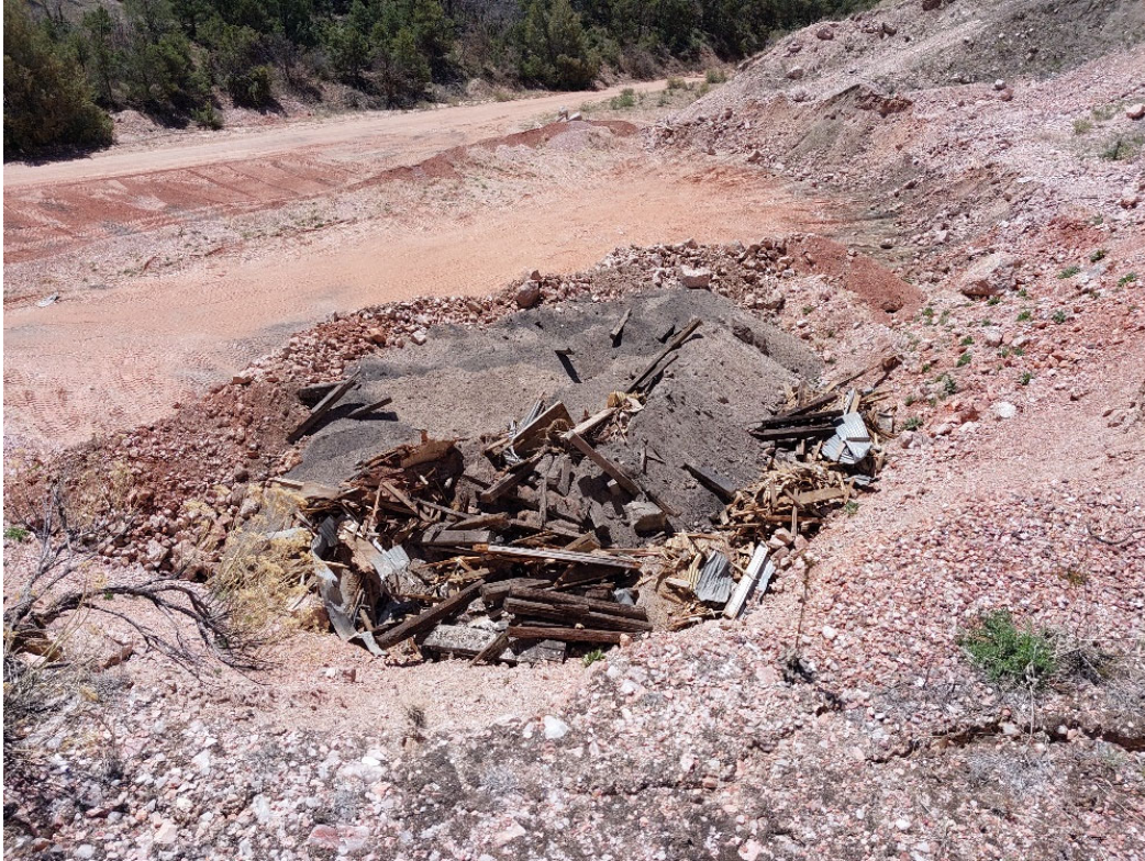
Photo #9: Sheet metal and lumber debris from an old pre-law structure that was demolished being used as backfill material. The lumber needs to be removed per the corrective action given at the beginning of this report.
