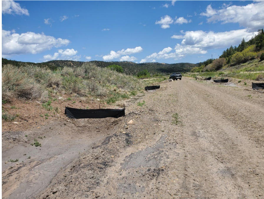
Photo 2: Some of the silt fences at the SAE south of Pond 007A.
