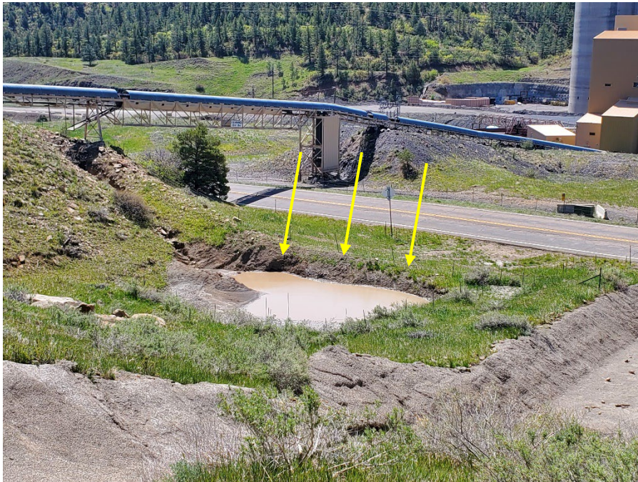
Photo 1: Containment #5. Arrow points to area where an excavator was recently used to remove sediment from the pond.
