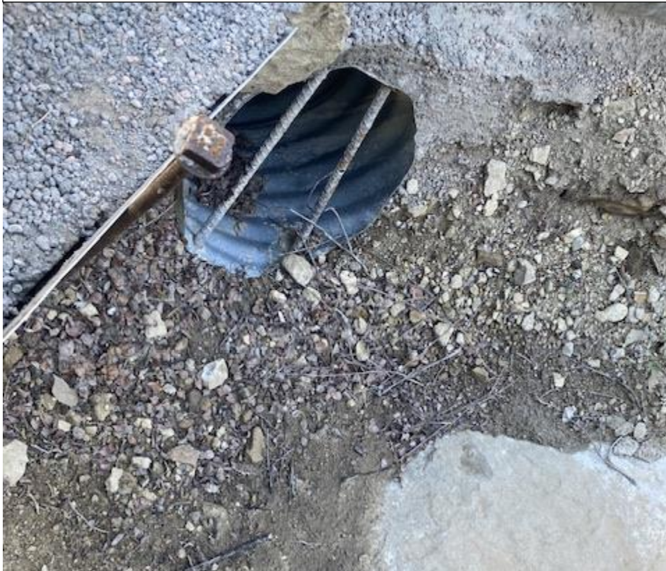
Photo 9: The inlet to the Sump E culvert.
