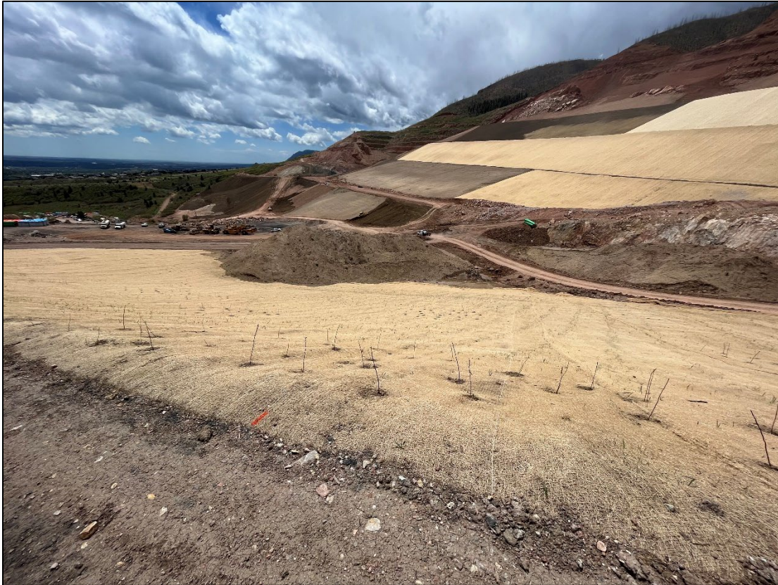
Photo 11: View southwest of tree and shrub planting in the north borrow area, topsoiling and matting efforts on the first four benches is also visible.
