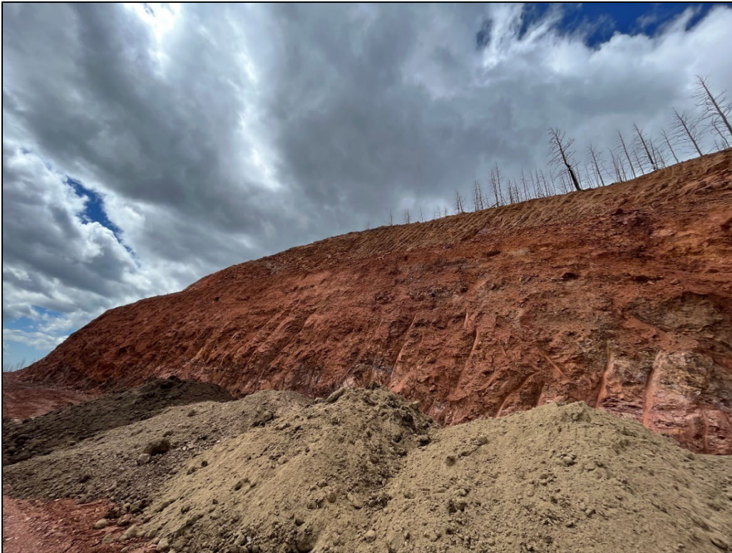
Photo 2: View north of final south peak highwalls, material has been placed on the bench in preparation for final topsoiling.
