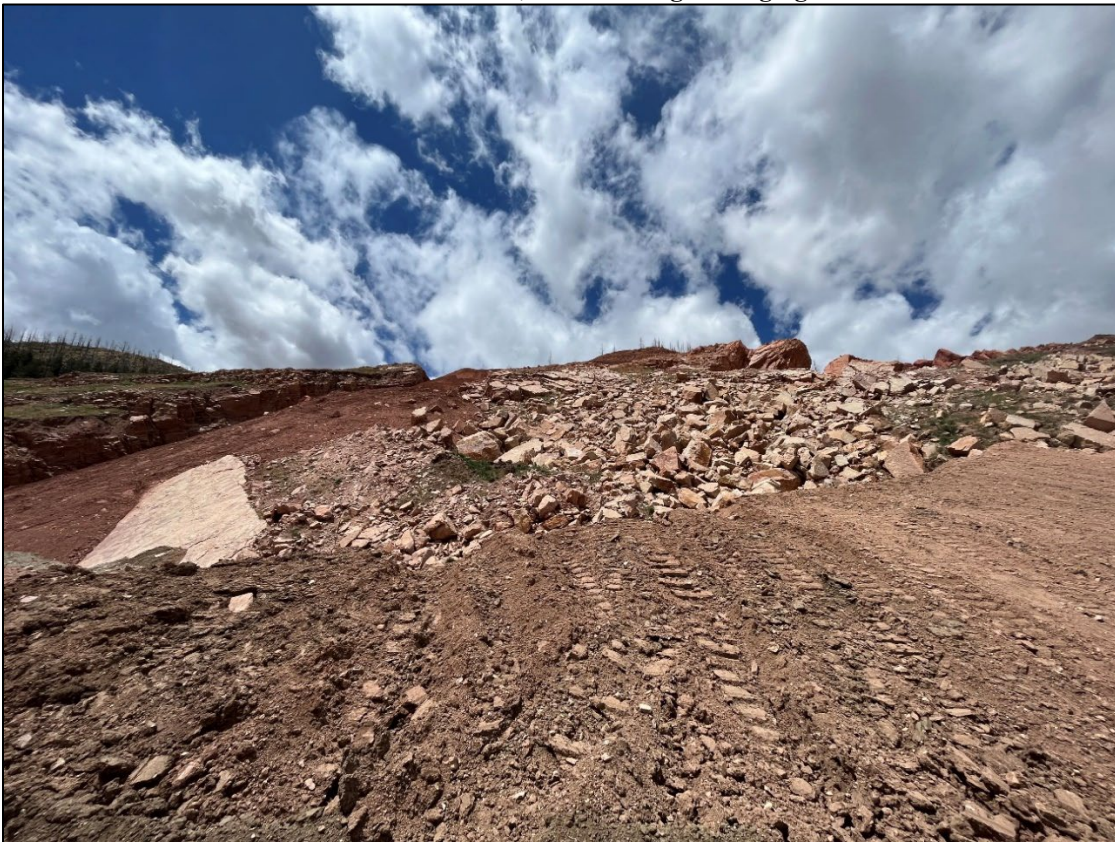
Photo 10: This slope, located to the west, will be partially filled in as a 2H:1V slope; some of the rocky material will remain partially exposed to allow for Bighorn sheep and other wildlife habitat.
