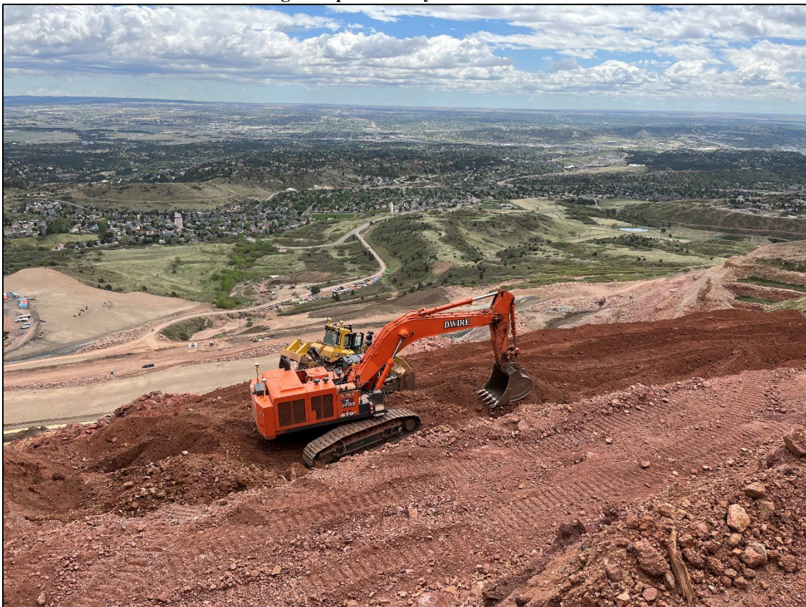
Photo 4: Excavators and dozers are working on the upper slope fill.
