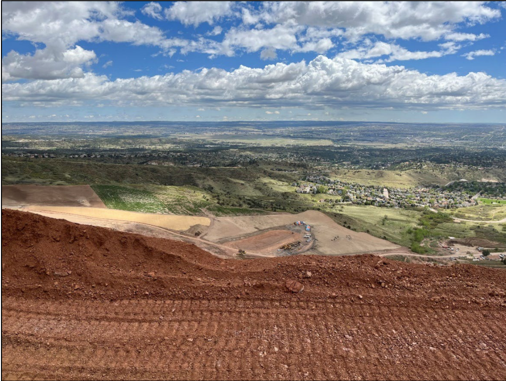
Photo 1: View east of the shop borrow area, currently receiving minimal backfill.
