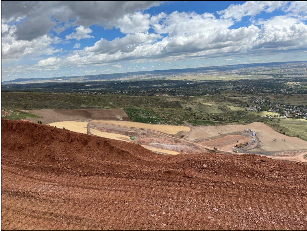
Photo 3: View northeast of the recently topsoiled, seeded, and matted northern area, the recently blasted 'Dragon's back' area is also visible along with preliminary cuts for the main north ditch.
