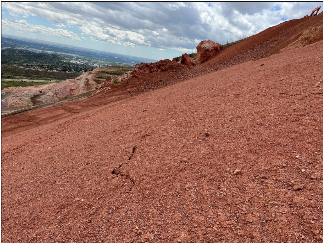
Photo 8: View south of the first crack on the upper fill slope.
