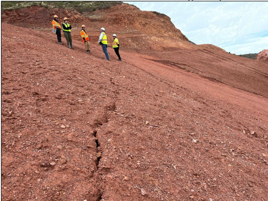
Photo 6: View north of the first crack noted on the upper fill slope; this was the deepest crack noted on site.
