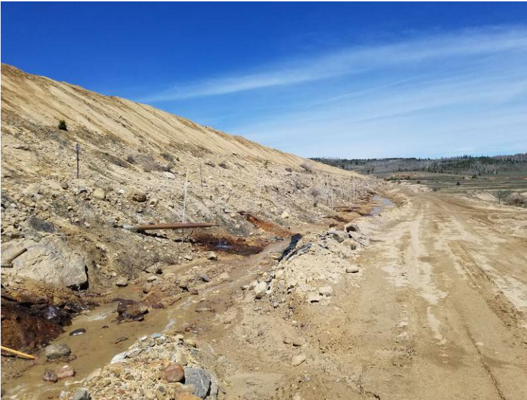
Figure 8. Toe of 1 Dam. Horizontal drains discharging into the seep water collection system.
