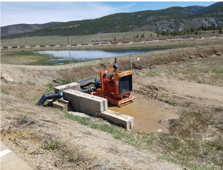
Figure 9. Back-up diesel pump staged and ready for the Ute Park Pump Station.
