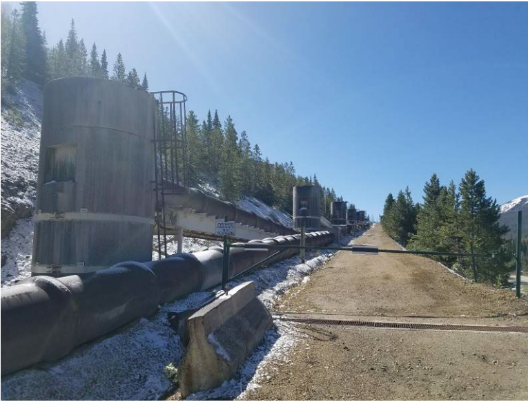
Figure 4. TDL and Emergency Cutout Line observed east of the Mill.
