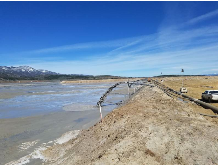
Figure 5. Active tailings deposition on 1 Dam crest.
