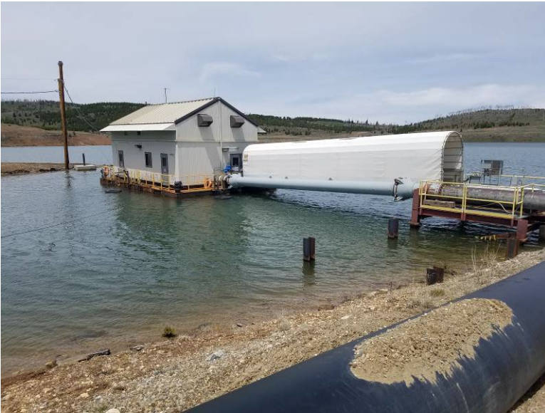
Figure 10. Barge Pump Station
