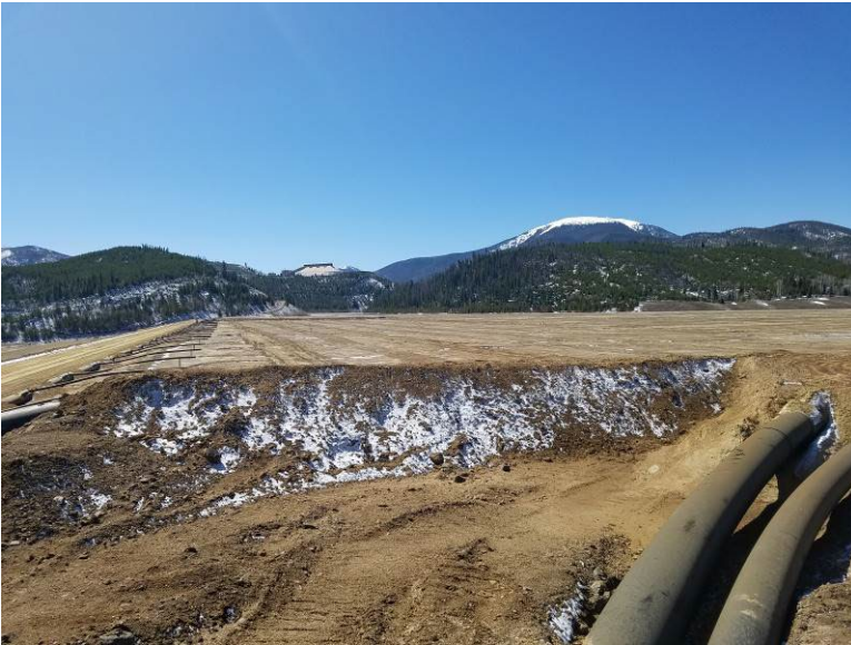
Figure 6. Top of 3 Dam. Treated for dust control.
