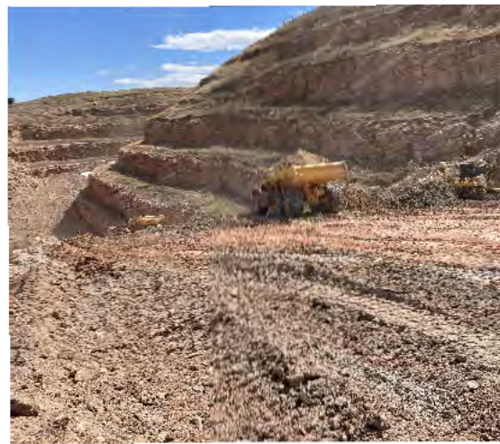
6. PLACING COMPACTED FILL ON BUTTRESS.
