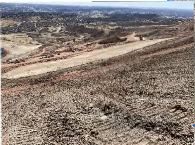
8. SLOPE BELOW CRACKING AREA. NO SIGNS OF MOVEMENT.
