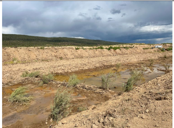
Photo 38: 8/25/2022 Completed SBS with direct transplants and willow transplants upstream and downstream of SBS.
