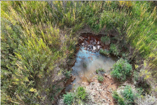
Photo 43: 9/18/2023 Headcut treatment completed in the southern headcut.
