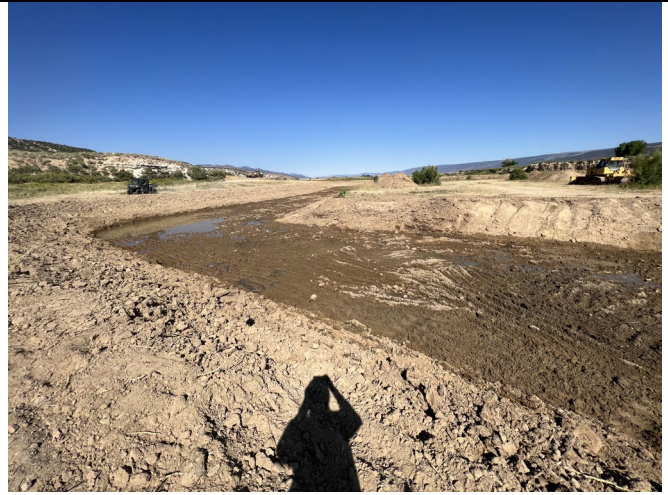
Photo 34: 8/18/2022 Completed channel excavation grading in upper reach.
