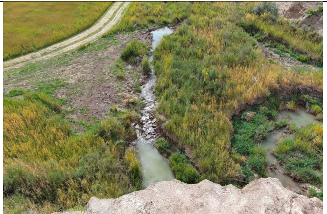
Photo 44: 9/18/2023 Headcut treatment in completed the northern headcut.
