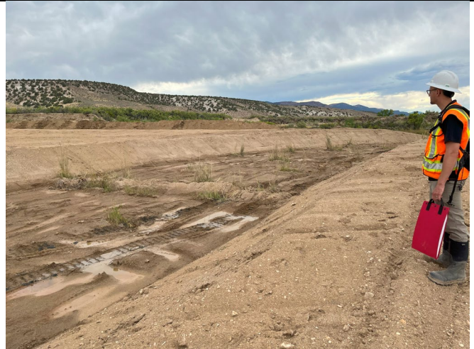
Photo 36: 8/25/2022 Completed SBS with direct transplants and willow transplants upstream and downstream of SBS.
