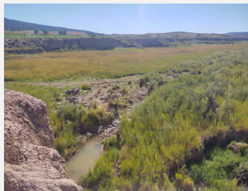
Fig. 16. Rock grade control installed at the top of the head cut.
