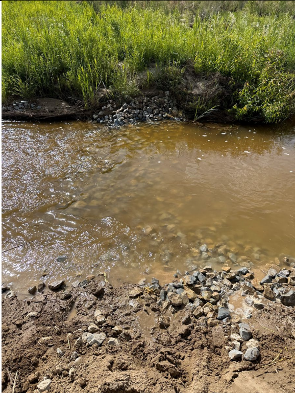
Photo 15: 6/16/2023 Downstream Check Dam BMP repaired
