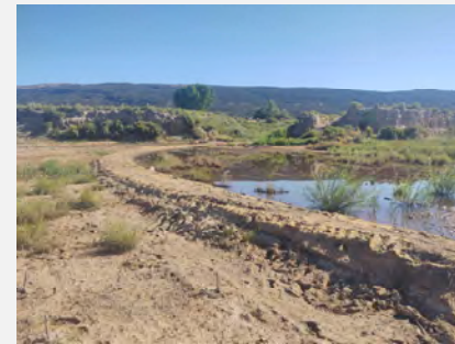
Fig. 24. Two photographs showing the berms partitioning wetland cells.
