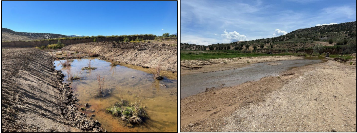
Figure 1. Post-construction channel (left photo) was SEM stage 2 (Channelization). Note the trapezoidal channel shape with no defined channel. SBS and transplants were installed to create disturbance including bank erosion to help push the channel further along the evolution trajectory. Post-flood channel (right photo) has widened and aggraded, moving towards SEM between Stage 5 and 6.
