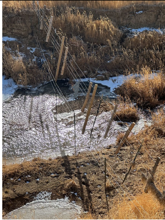
Photo 50: 12/17/2023 Fence extenders to preclude cows from entering site
