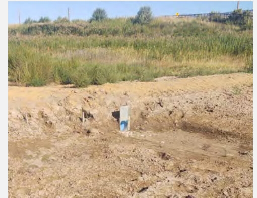
Fig. 27. The berms creating the wetland cells are pierced with a plastic pipe, fitted with a flow control gate that can be pulled up to increase flow volume.
