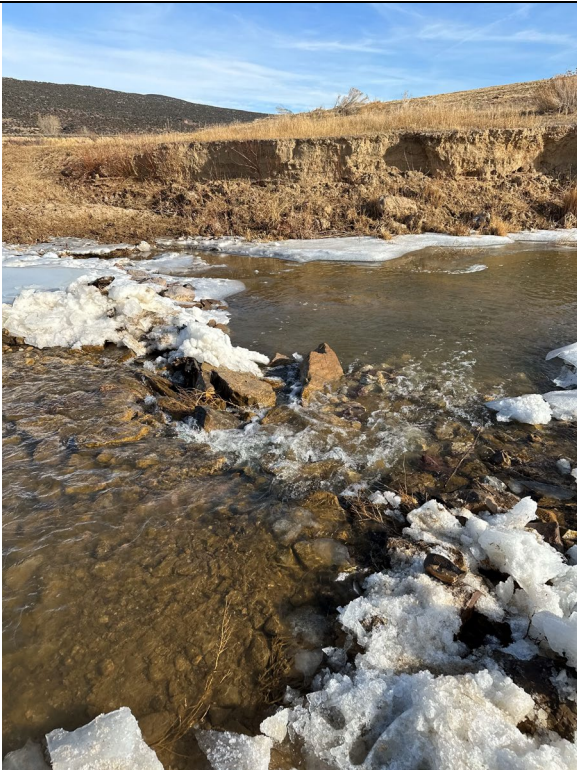
Photo 51: 12/17/2023 Added native cobble to upstream low water crossing to reduce fish passage barriers.
