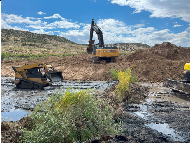
Photo 33: 8/17/2022 Completed channel excavation grading in lower reach.
