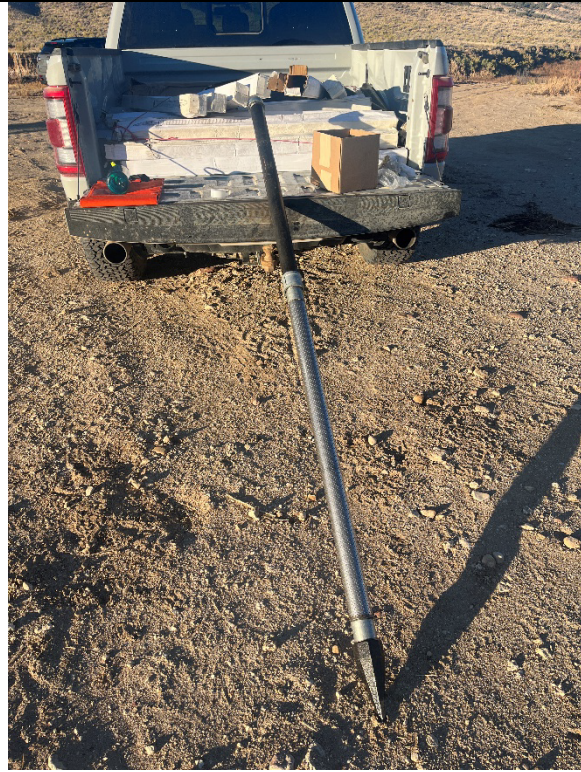
Photo 46: 10/17/2023 Assembled Drive Point Groundwater Well before installation.
