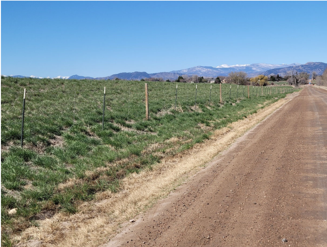
Photo 20: View of the vegetated overburden berm and barbed wire fence running along the northern edge of the permit area.
