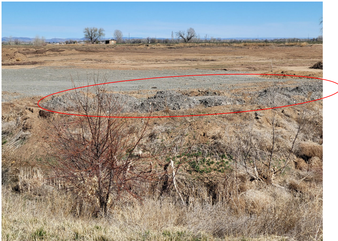
Photo 10: Closer look at inert fill in Cell C. Stockpiled imported material circled.
