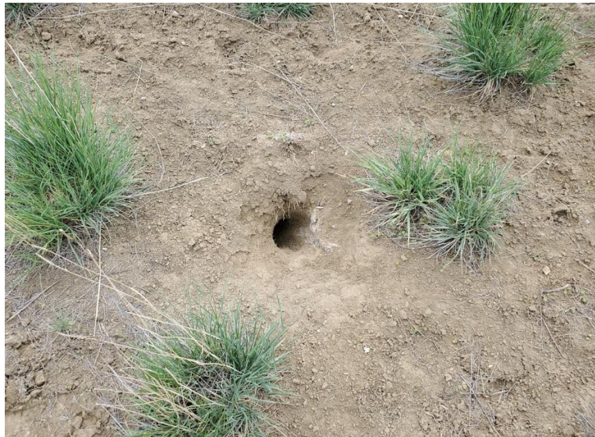
Photo 8: View to the southeast of animal burrow in the RP-4 Pond embankment.
