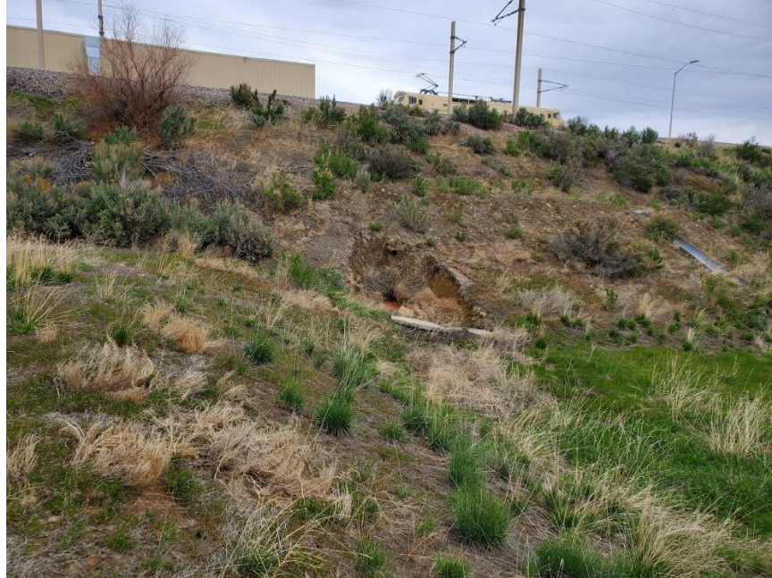
Photo 5: View to the north of erosional scar in the Rail Loadout Pond. The scar does not appear to have grown in size.
