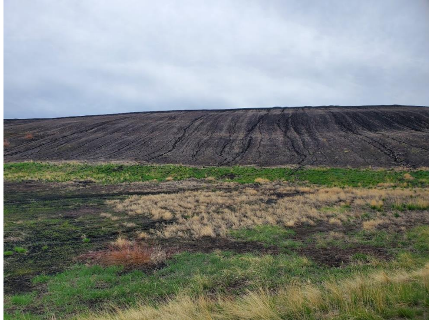
Photo 7: View to the south of rills that have extended into the RP-4 Pond.
