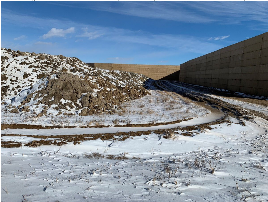
Photo 10 – Sediment control ditch on southwest corner of Area C.
