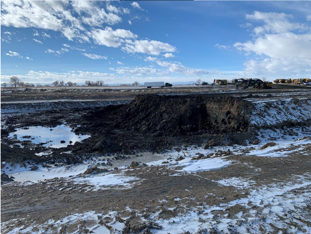
Photo 1 – First layer of material being removed. Excavation will continue deeper once water level is lowered.
