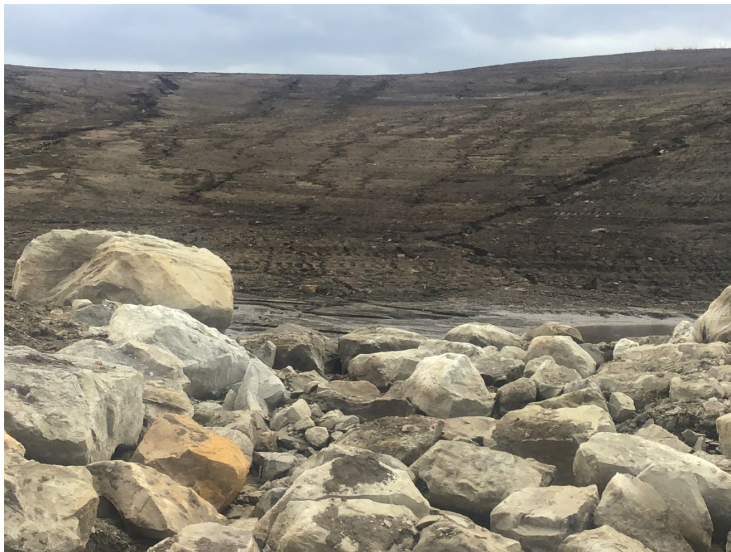
Photo 14: Rills on northwest facing slope of D Pit.
