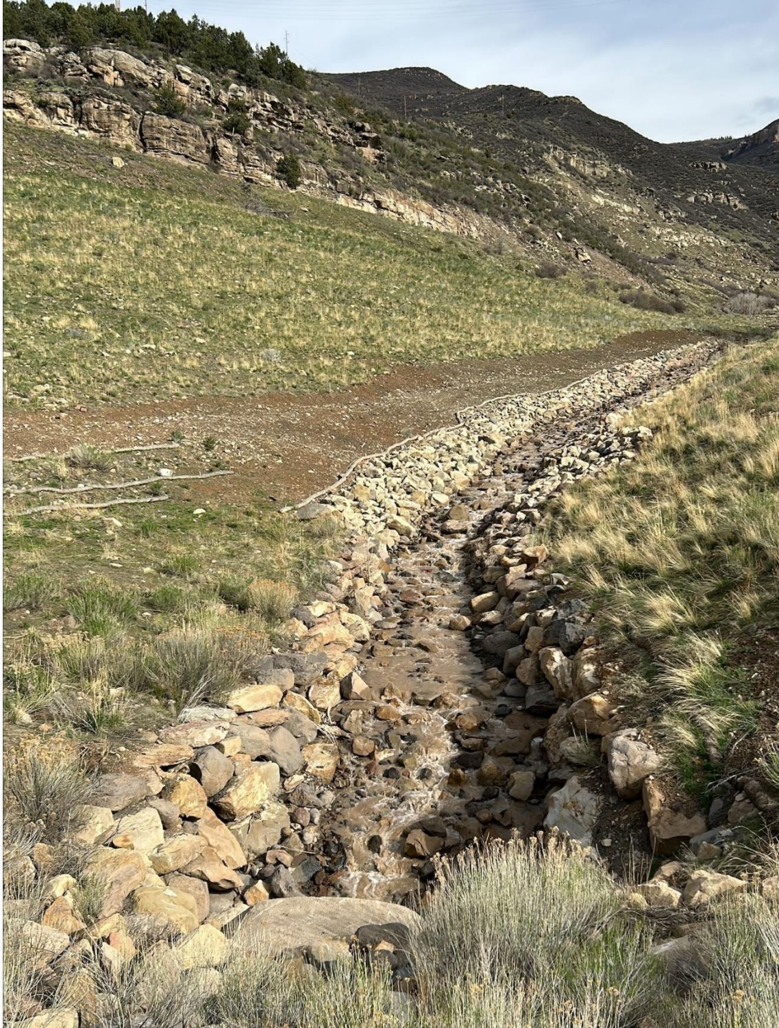
Figure 1: Lower section of Elk Creek channel, with repair on left bank
