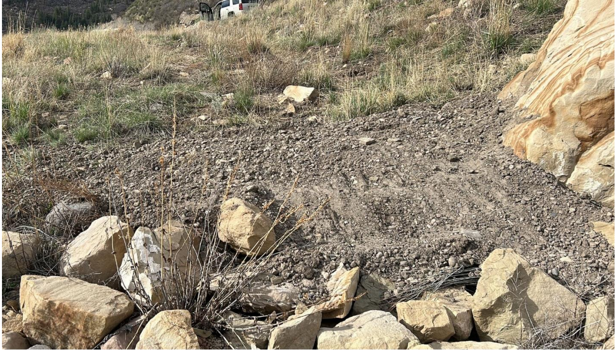
Figure 5: Repair to backfill around inlet to middle section of Elk Creek culvert
