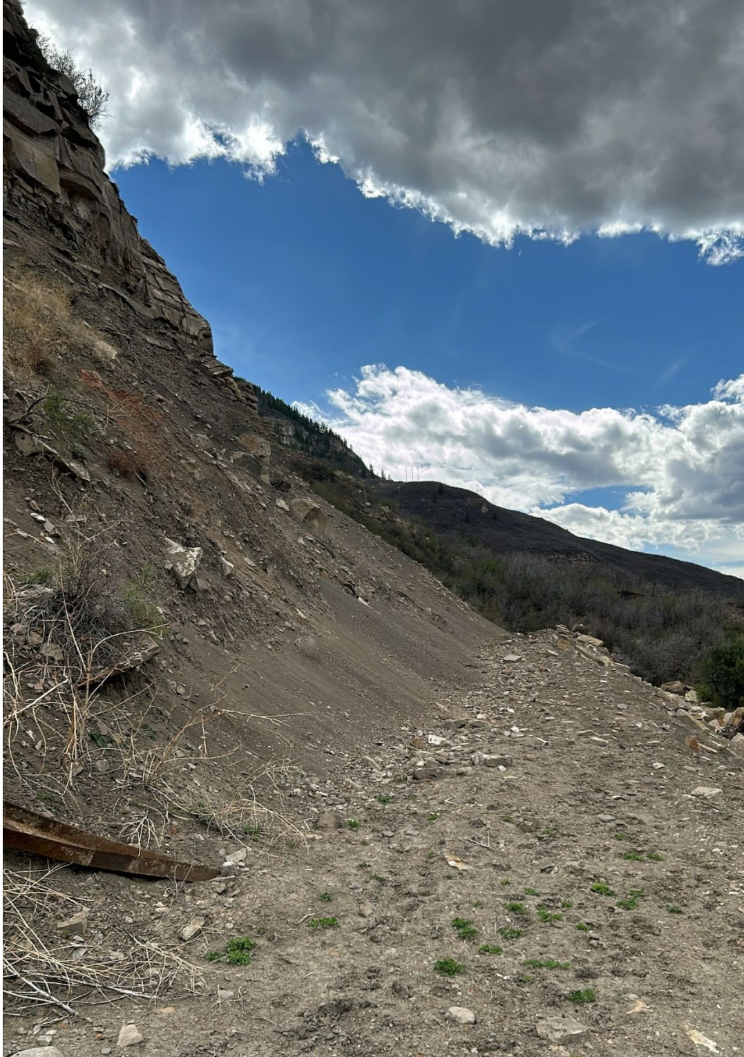
Figure 7: Road below scarpe, showing accumulation of spalled material
