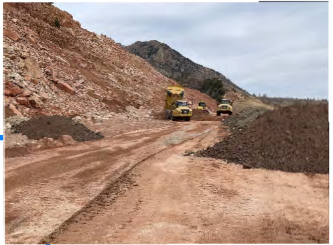
3. HAUL TRUCKS PLACING FILL ON BENCH.
