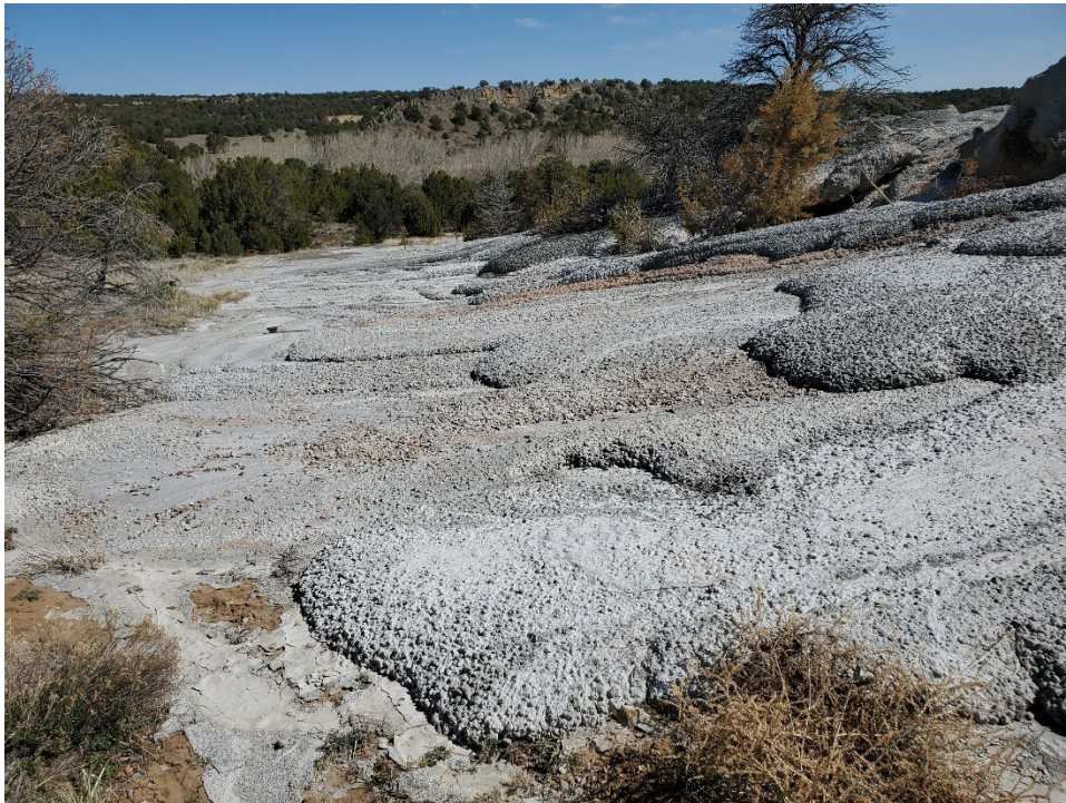
Photo 4: Looking downslope at the concrete washout.
