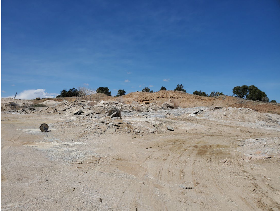
Photo 5: Looking north-west at the concrete/equipment storage area within the permitted boundary that's part of the lease agreement.
