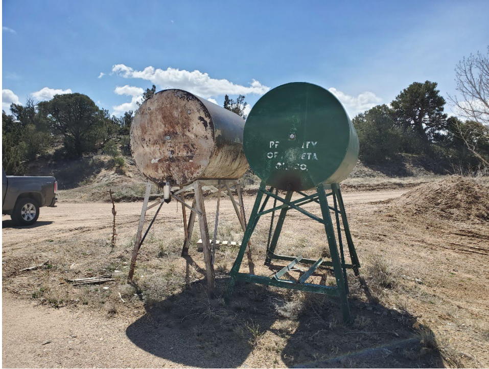
Photo 1: Fuel tanks that will require secondary containment if they are to be used again.
