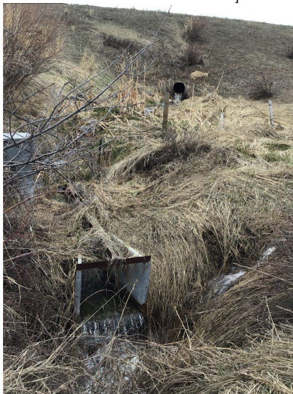
Photo 2: Pond 12 decant culvert and weir
