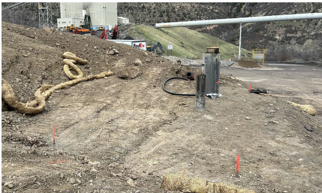
Figure 22: Cased borehole and stakes for concrete pad
