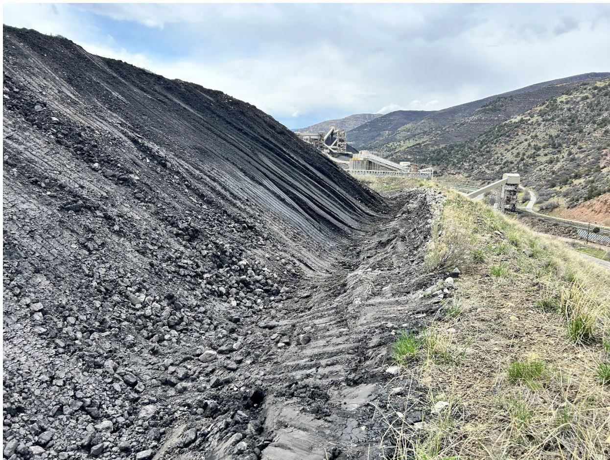
Figure 28: Work in progress to improve drainage on LRP (Photo 2 of 4 from MCC)
