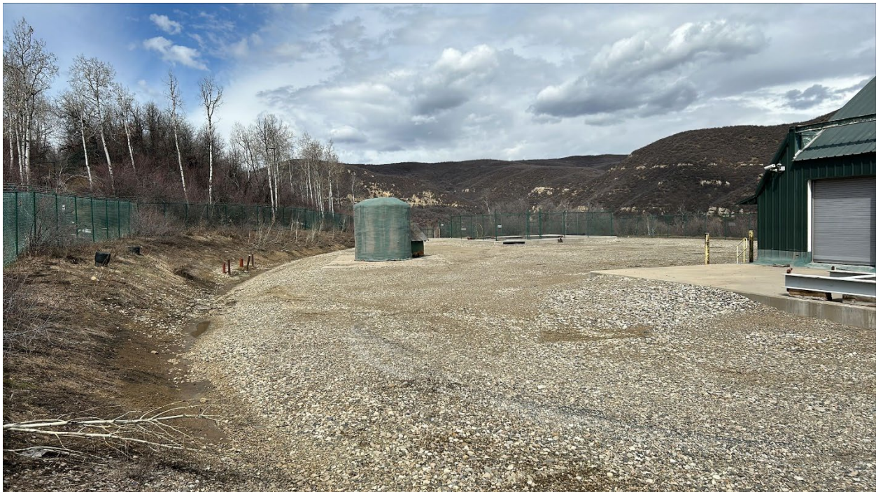
Figure 4: Graveled pad with positive drainage and sediment control
