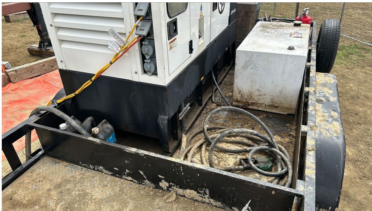
Figure 12: Secondary containment on generator trailer
