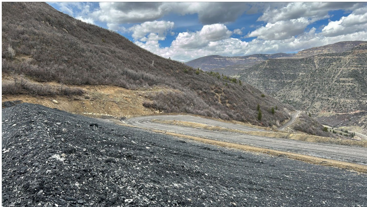
Figure 18: Compacted face of RPEE, with top of haul road
