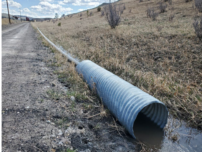
Photo 7: Ditch D2 being used to pump water from Pond 006A to Pond 004.
