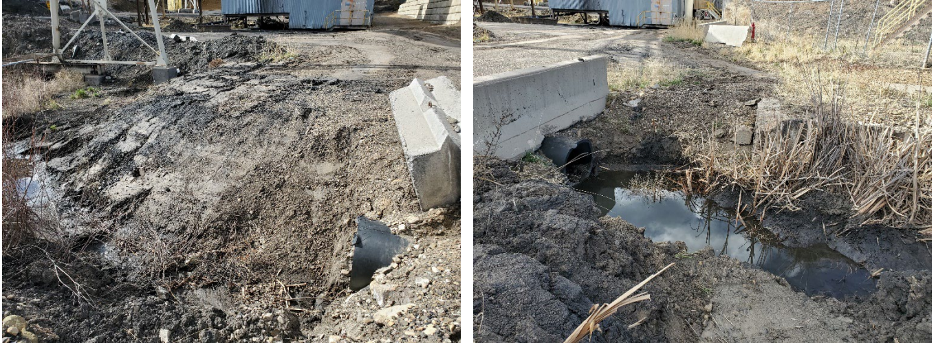
Photo 3: (Left) Stabilized bank around C16D. (Right) Cleared out west side of C16D.
