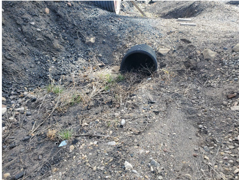
Photo 8: C17A has accumulated excess sediment.
