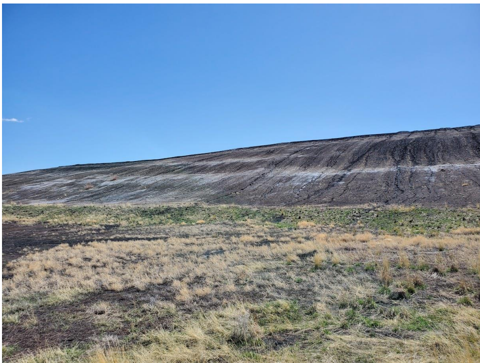
Photo 8: View to the southeast of rills on RP-2/3/4 pile that extend into Pond RP-4
