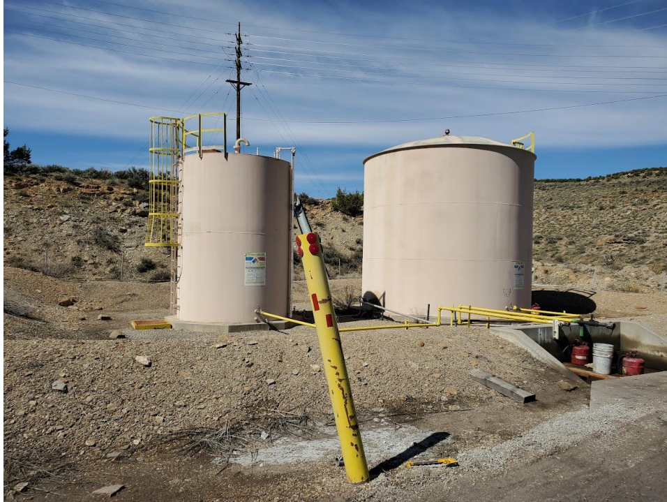
Photo 9: View to the east of fuel tanks in secondary containment.
