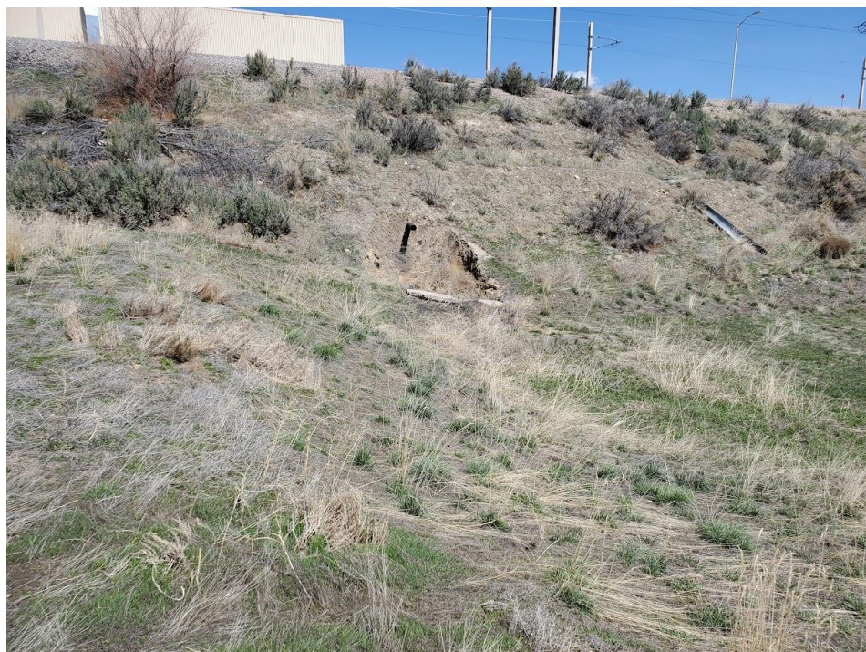
Photo 6: View to the north of erosional scar on Pond RP-1. Does not appear to have enlarged.
