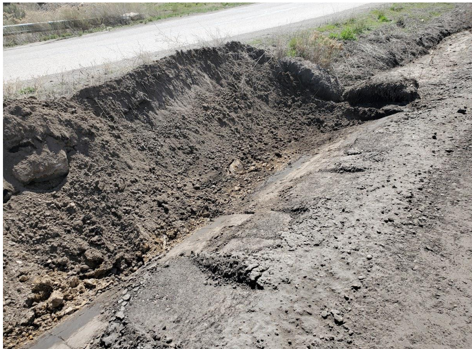
Photo 10: View to the southeast of conveyance ditch along haul road. Crews have cleaned sediment from the ditch.
