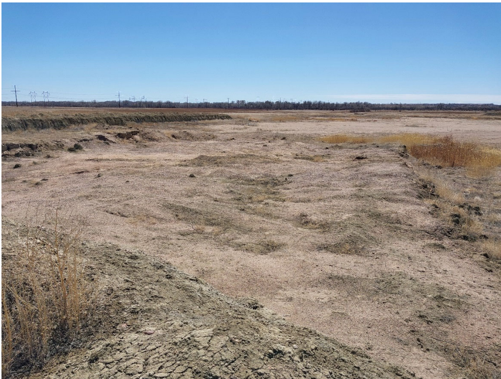
Photo #8: Backfill and grading done east of the largest pond.
