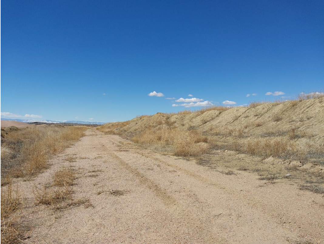
Photo #9: Haul road along the north side of the permit boundary, berm to reduce noise and visibility effects and support stormwater management plan on the right side of the road; photo taken looking to the west.
