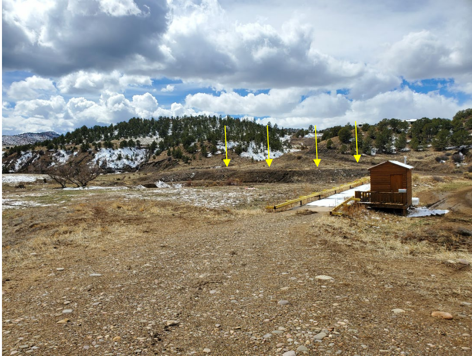
Photo 3: Arrows point to the 'Reclamation Only' area within the creek bed. This area has not been re-disturbed since it was reclaimed.
