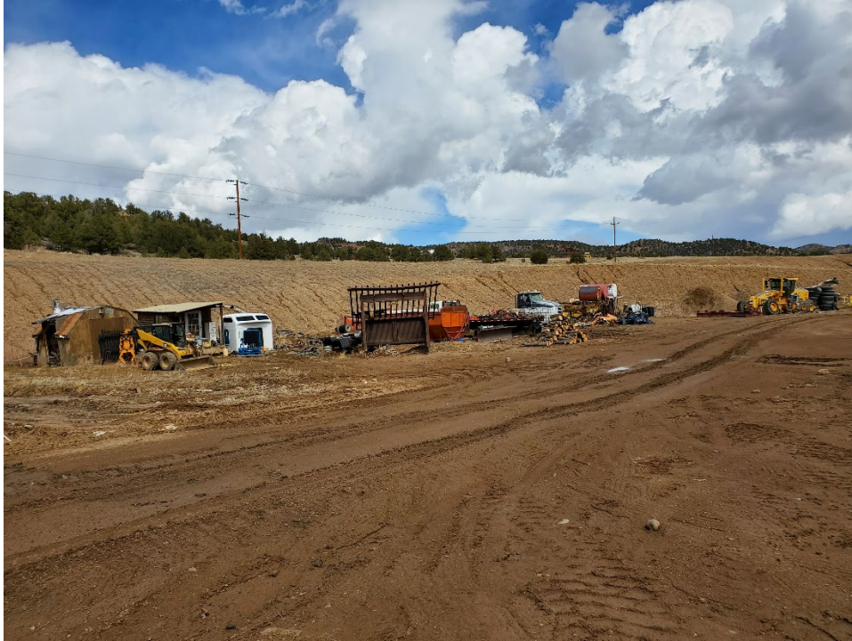
Photo 11: Looking north-east along the reclaimed slopes, and some of the equipment stored, in Area 1.
