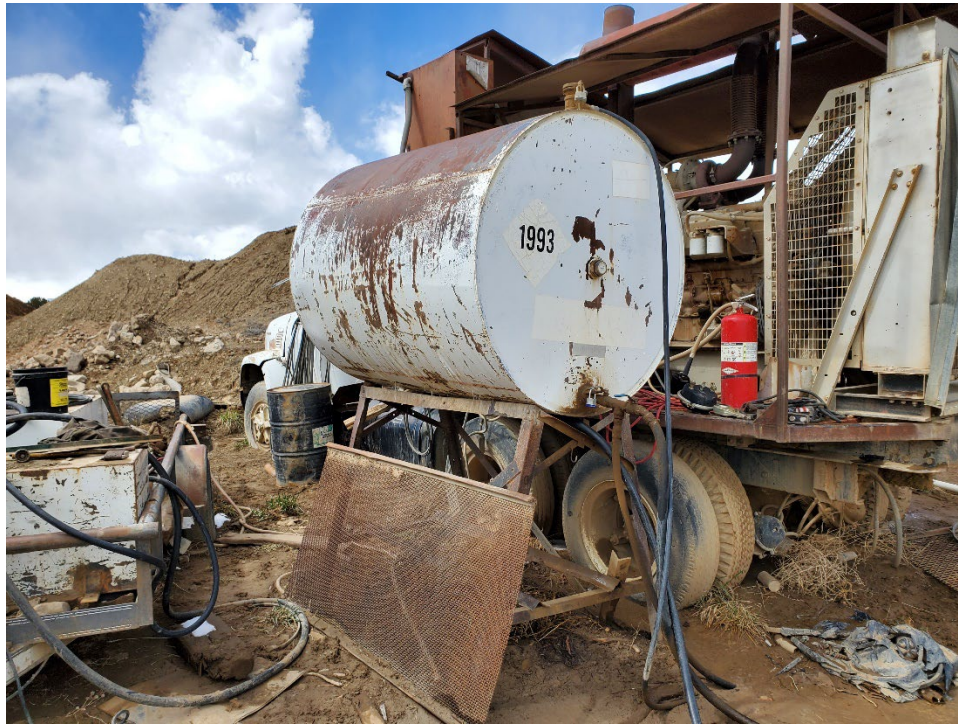
Photo 1: Fuel tank in Area 1 requiring secondary containment.
