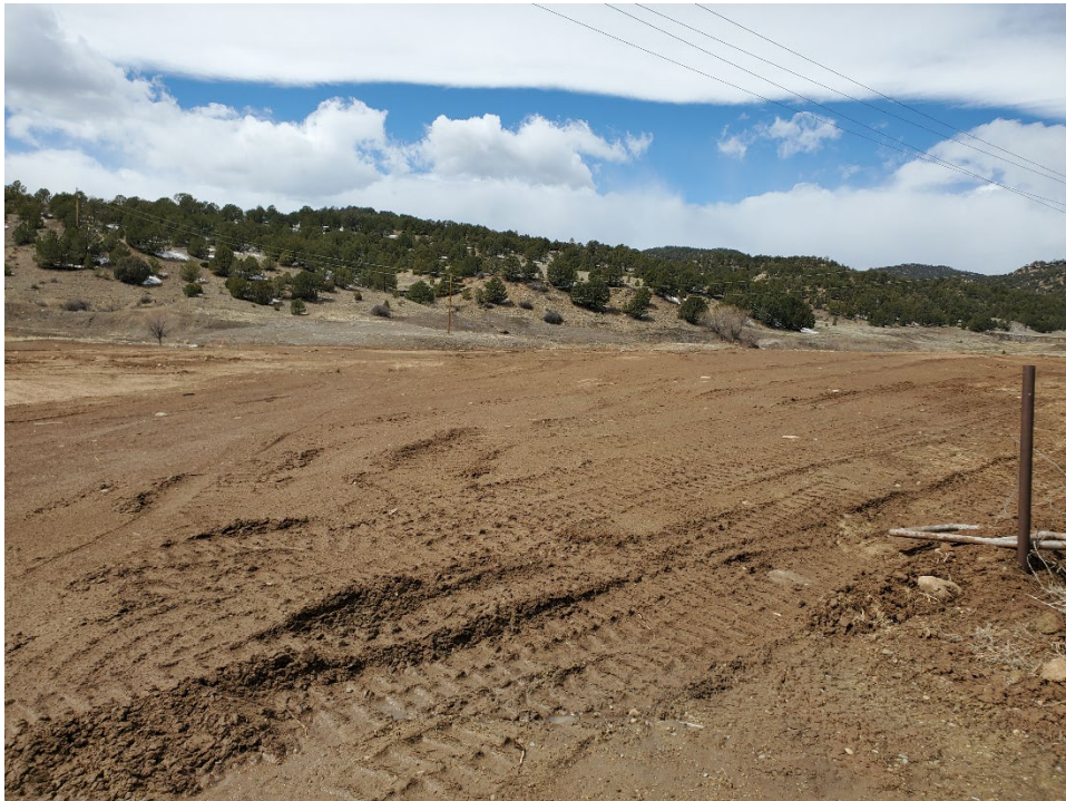
Photo 4: Standing at the north side of the entrance road, looking north-west at the widened embankment on the north-portion of the entrance road.
