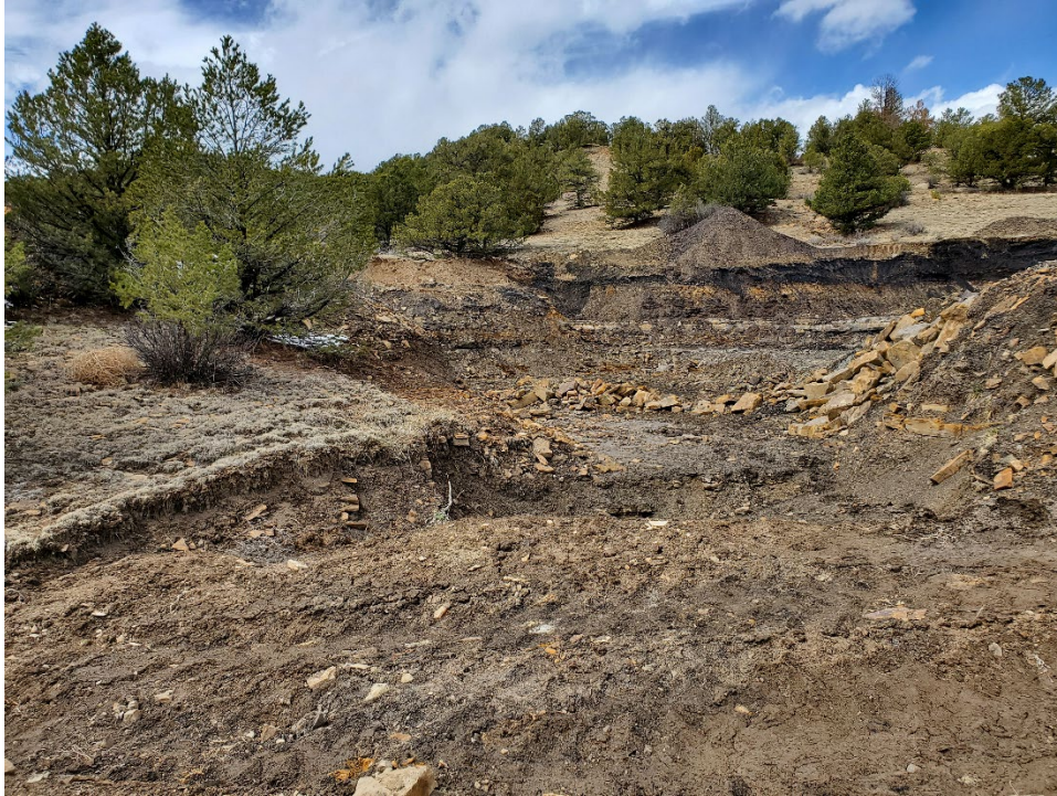
Photo 19: Looking north-west into the pit area in Area 3.
