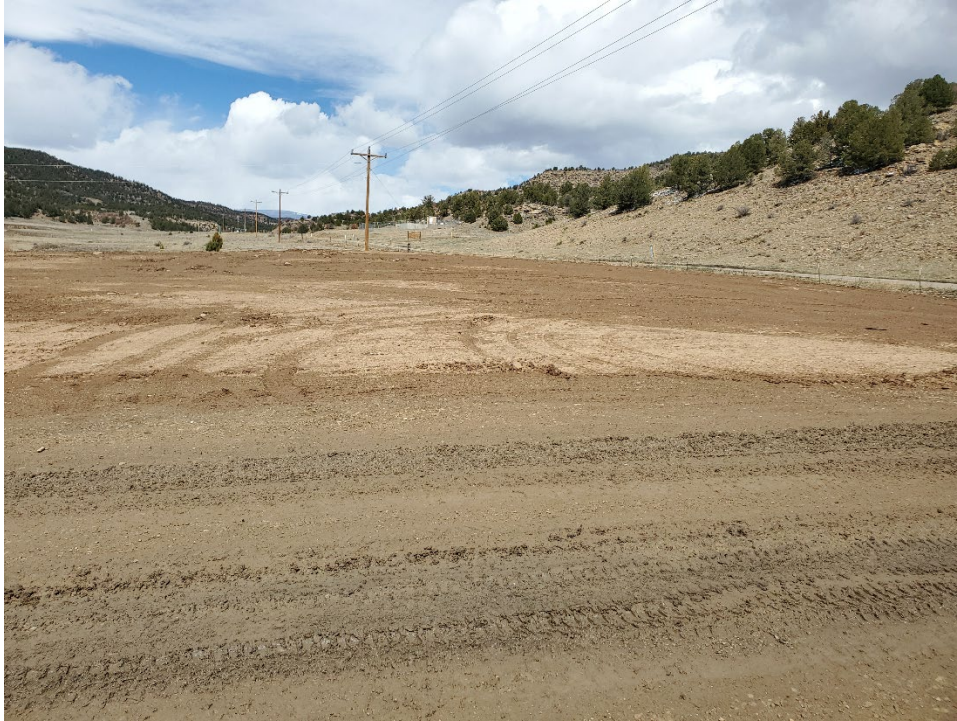
Photo 5: Looking north across the widened embankment on the north-portion of the entrance road.
