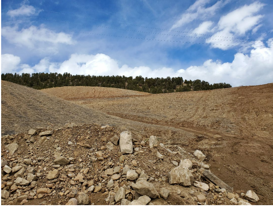
Photo 25: Looking north-west at some reclaimed slopes. Some rilling is seen on the slopes.
