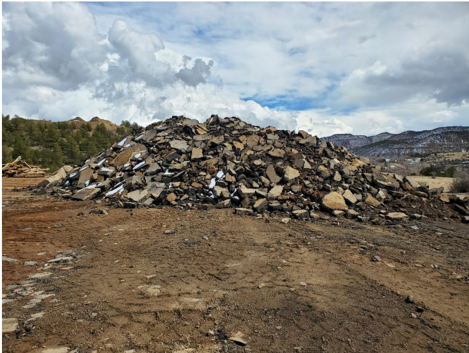
Photo 14: A pile of broken up asphalt from a bridge demolition, brought into the pit to be crushed and combined with product.
