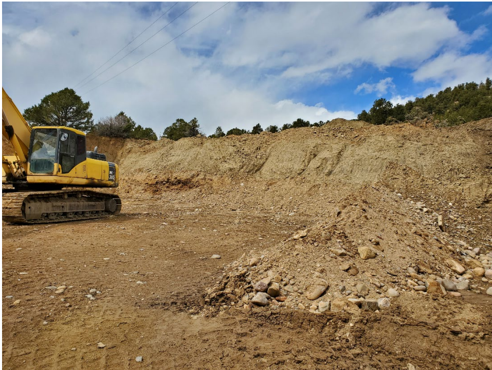
Photo 10: Looking north-west at the start of the highwall on the east side of the northern pit of Area 1.
