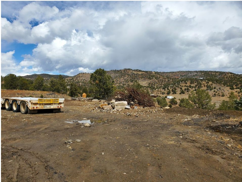
Photo 18: Facing north-east, looking at a pile of rebar/scrap metal salvaged from a bridge demolition. Pile is being stored until it can be hauled off-site.
