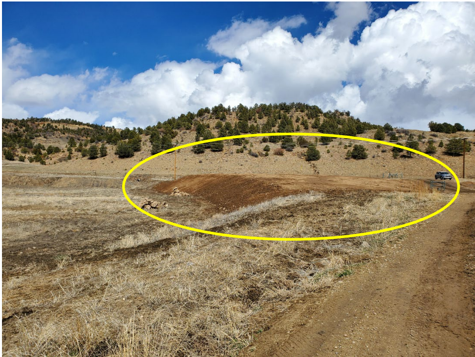
Photo 6: Looking east at the widened embankment on the north-portion of the entrance road (circled).
