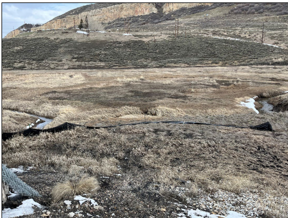
Photo 10: View west towards Foidel Creek taken from behind the stoker loadout building, silt fence is in need of repair.
