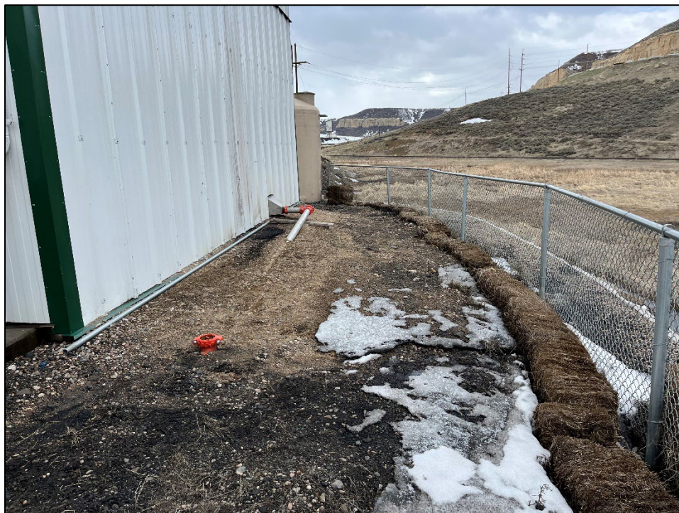
Photo 11: Hay bales behind the loadout building need to be replaced.
