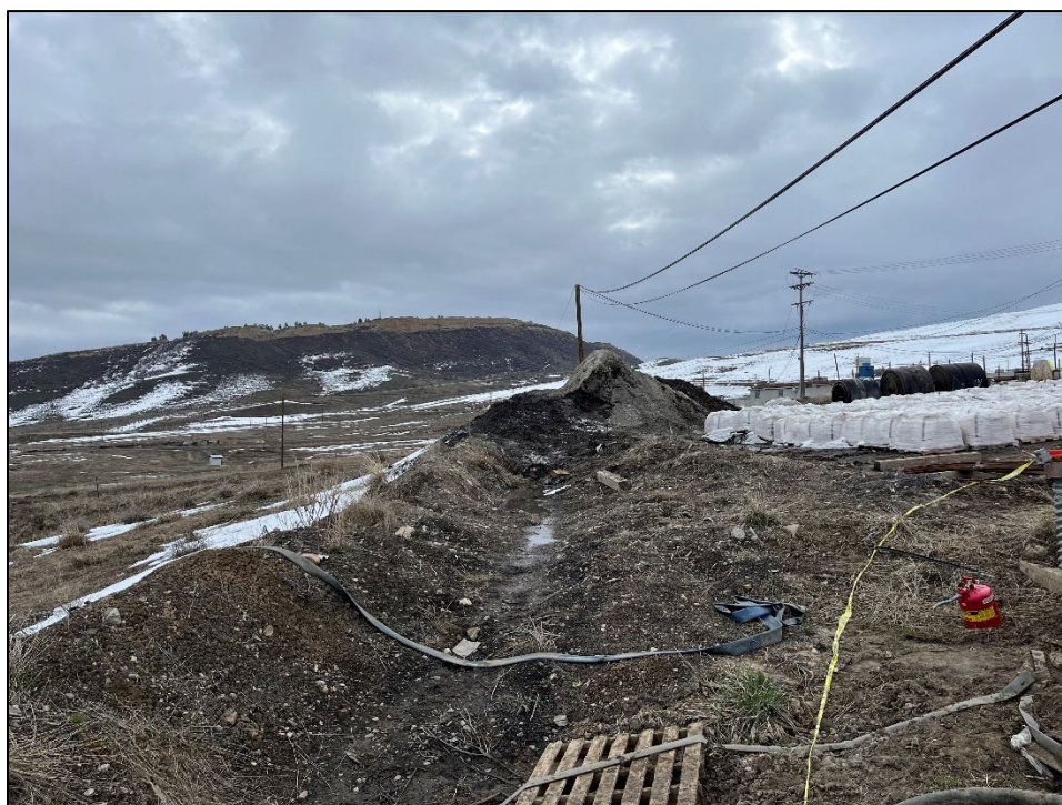
Photo 6: Remnants of snow, ice, and debris have been pushed into the ditch located behind the warehouse, removal of this blockage has been added as a maintenance item.
