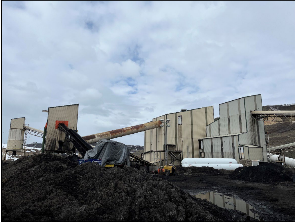
Photo 7: A temporary conveyor has been added to the wash plant facility.
