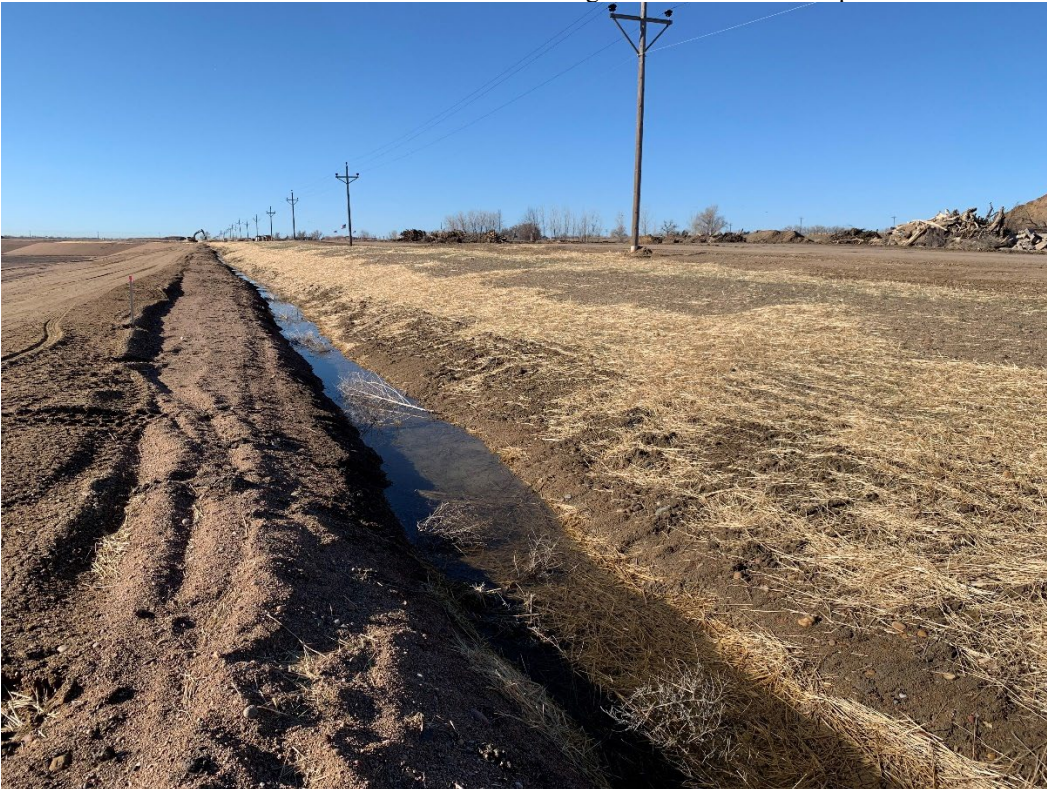
Photo 3 – Western side stormwater diversion ditch, water flows toward picture.
