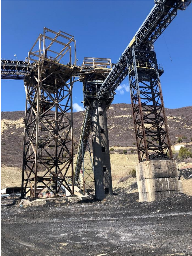
D Portal Bench – stacking tube and conveyor supports
