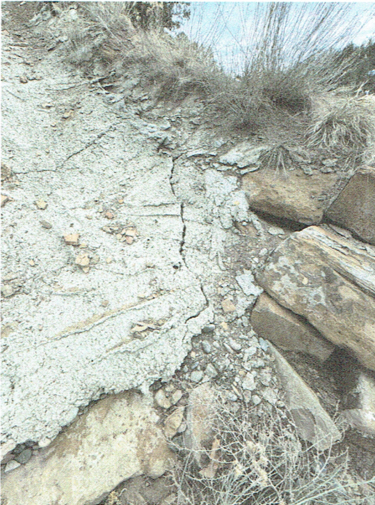
Pic. 2 – Minor cracking, lower armored section of Reach 1.
