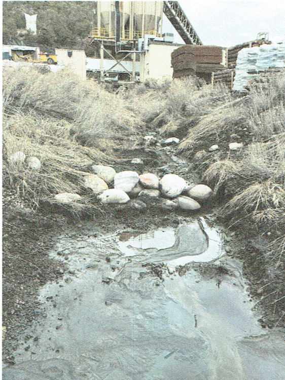
Pic. 3 Erosion control measures south of the scale house.
