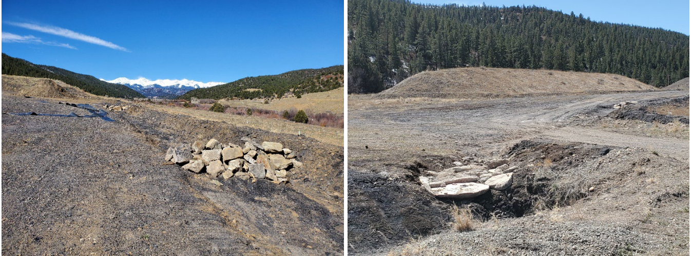
Photo 23: Check dams along both sides of the Stockpile Storage Area. The erosion has been repaired and the area has been stabilized.
