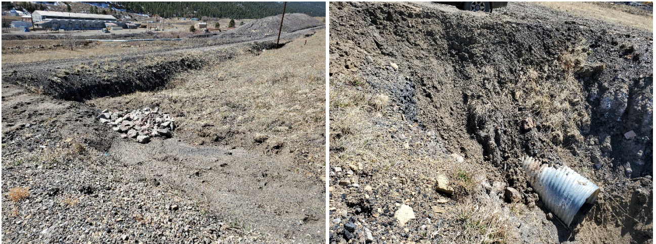
Photo 7: (Left) ground above C14. (Right) Bank repaired around C14.
