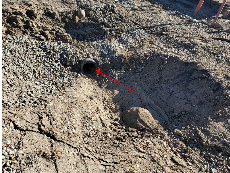
Photo 6: The arrow points to C12. The area around the culvert has been cleaned.
