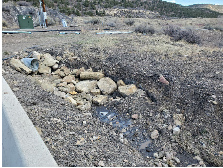
Photo 8: Repaired area around C65 that water had undercut.
