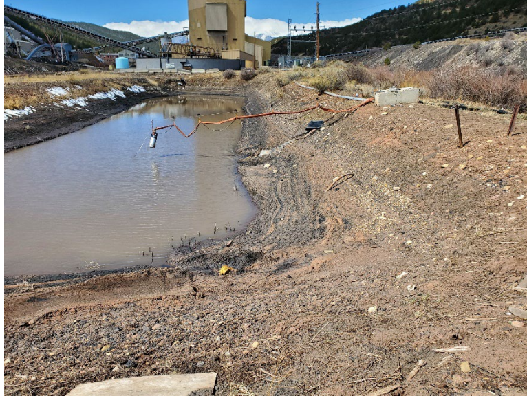
Photo 14: The north-east bank of Pond 006A, where water had begun to incise the bank, has been repaired.
