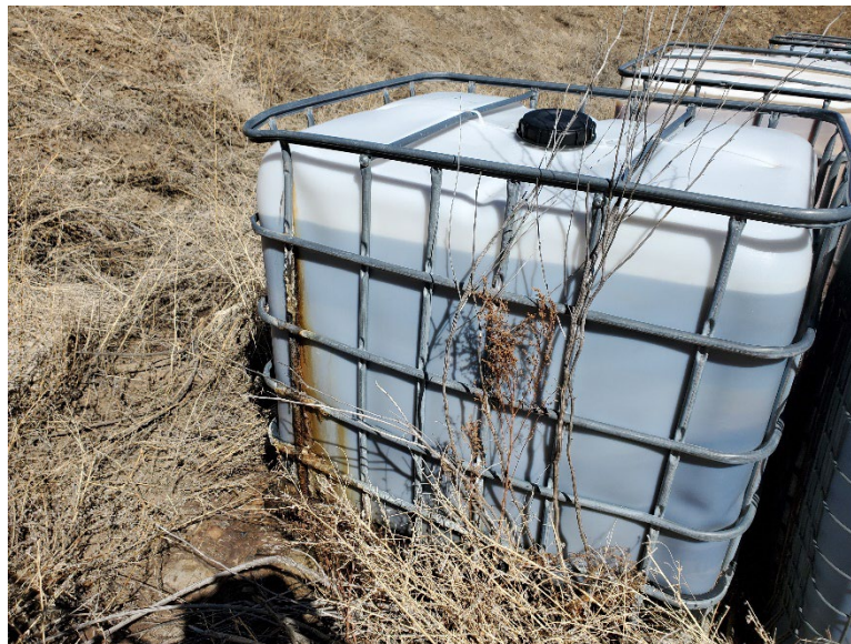
Photo 21: Leak observed on a mag-fluoride tank.
