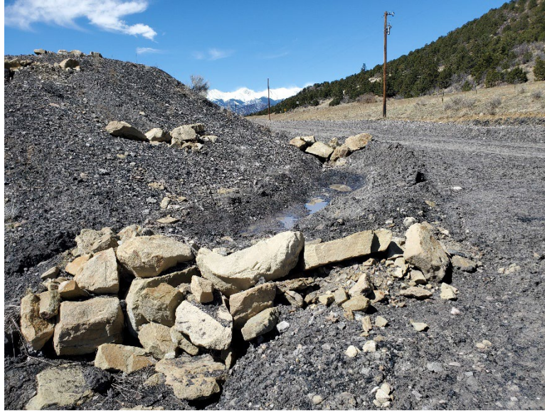
Photo 1: Check dams along north-east side of the DWDA #2.
